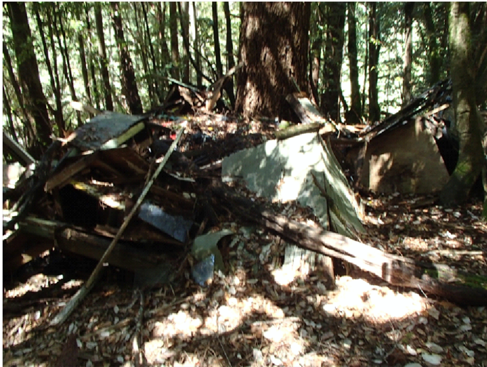
Collapsed Shed at ECDM
