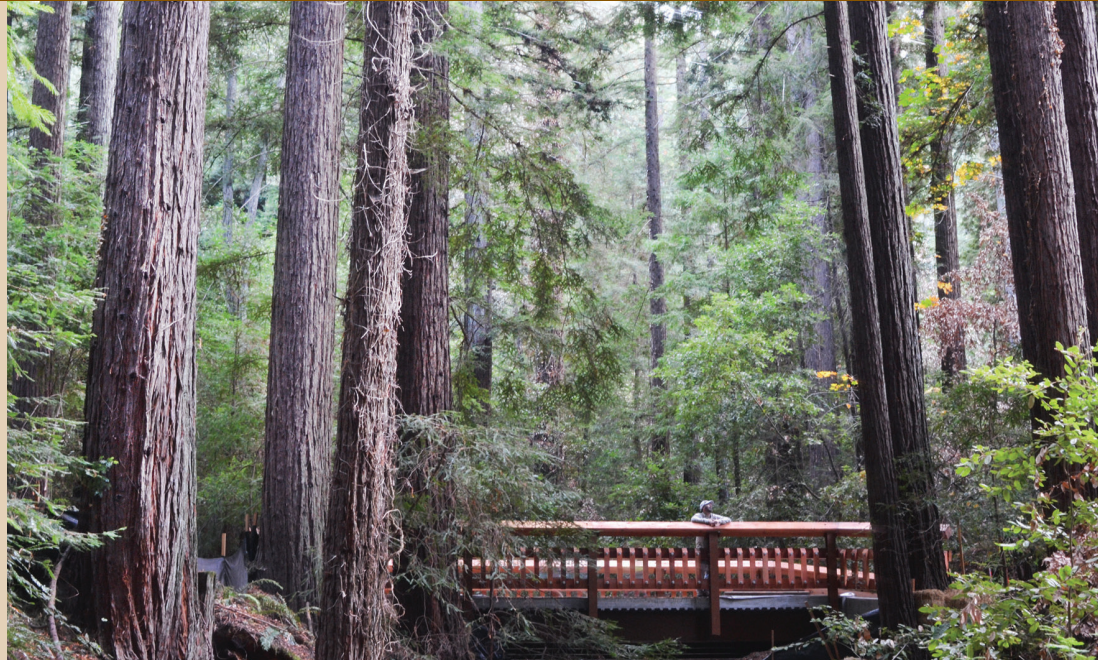
Under construction: A new trail and bridge over Webb Creek in Bear Creek Redwoods Open Space Preserve
