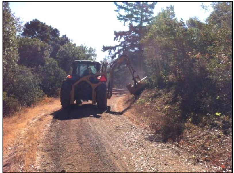
Figure 3: Preserve roads are maintained to allow safe passage of emergency vehicles
