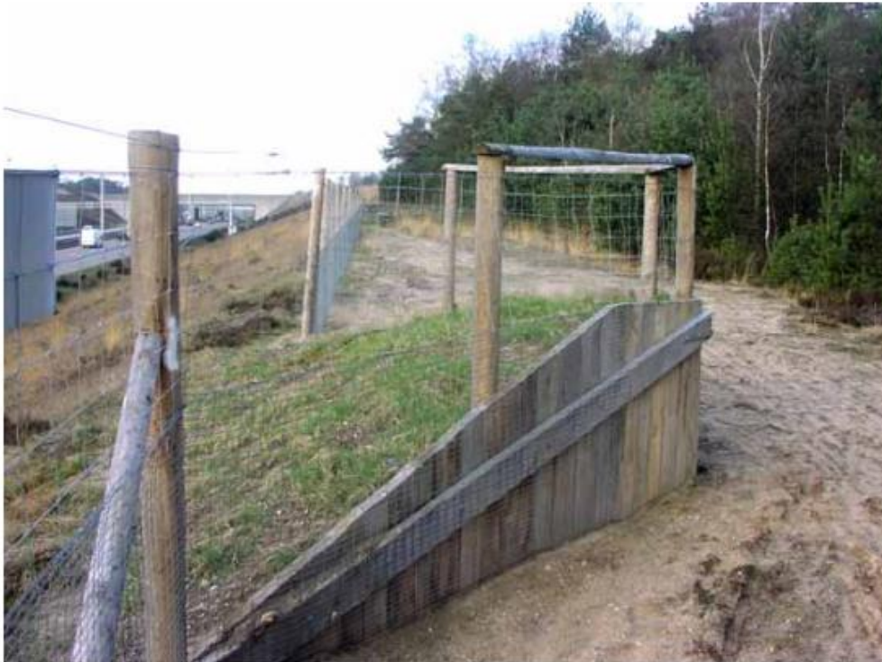
Figure 1.4-6: Example of a wildlife escape ramp (FHWA 2011). The height, color, and materials used for this project may differ
