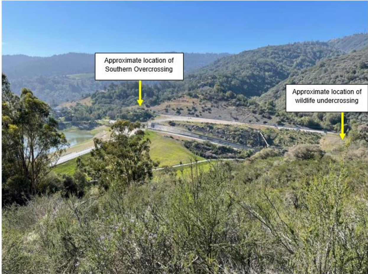
Figure 2.2.3-2: View of the southern and central project area, looking west/southwest from the Jones Trail; yellow arrows indicate approximate locations of the Southern Overcrossing and wildlife undercrossing
