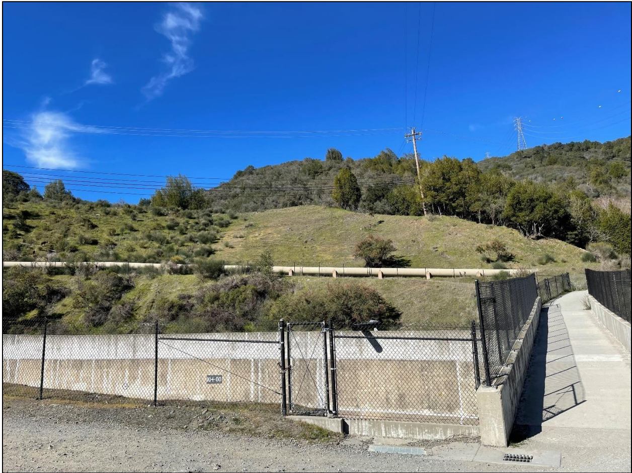
Figure 2.2.7-6: KV-2 Existing Condition/No Build Alternative
