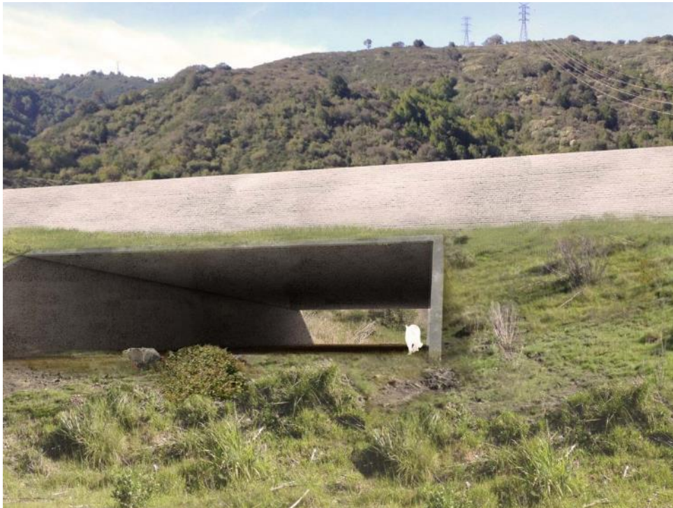
Figure 1.4-4: Simulated view of a concrete slab unit bridge, facing west toward the wildlife undercrossing and Trout Creek, below northbound SR 17 (Midpen 2019a)
