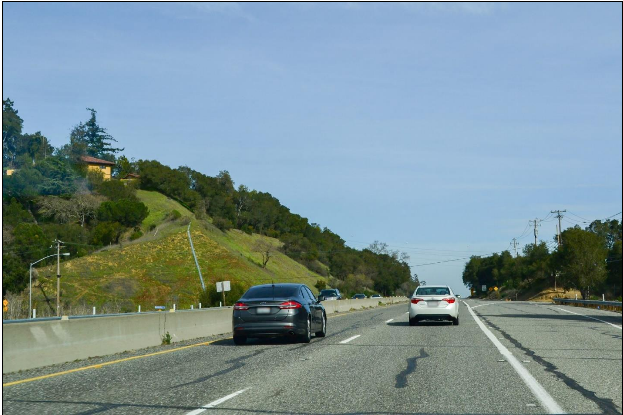
Figure 2.2.7-10: KV-4 Existing Condition/No Build Alternative
