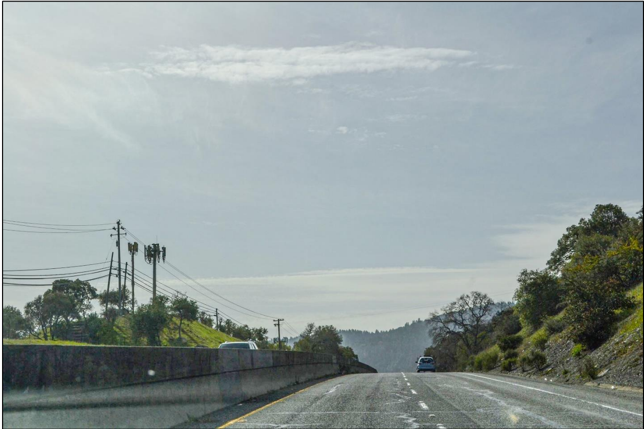
Figure 2.2.7-8: KV-3 Existing Condition/No Build Alternative
