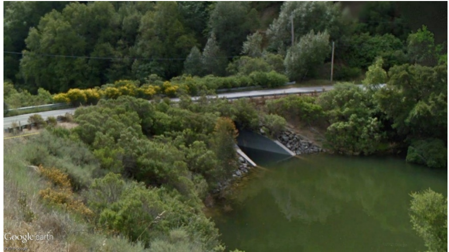
Type 3: Above large culvert at Limekiln Creek
