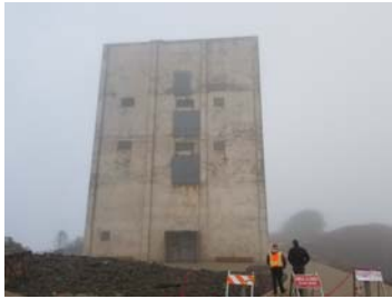
Radar Tower North Face
