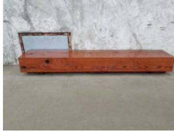
Bench Adjacent To Tower - with Paint Chips
