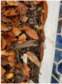
Ceramic Tile and Grout Old Pool Area
