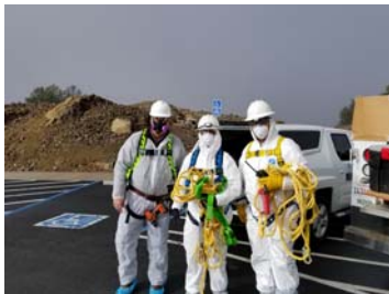
Fall Protection For Roof
