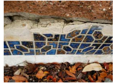
LEAD - HMS-M17224-04PB Ceramic Tile Glaze
