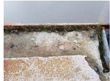
HMS-M17224-22A Roof Penetration Mastic - East Edge
