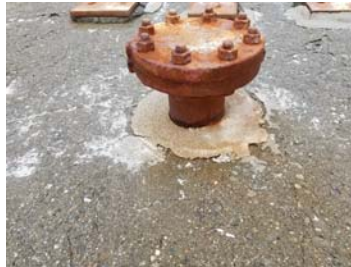
HMS-M17224-21 Penetration Sealant Cementitious
