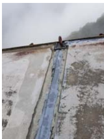
HMS-M17224-26A Mastic Under Single Ply
