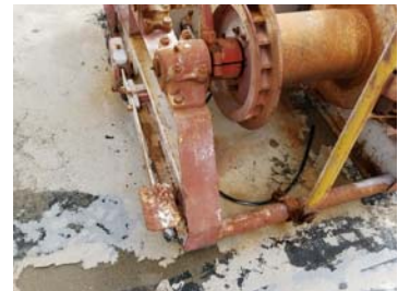
HMS-M17224-25A Roofing and Mastic at Gear Device
