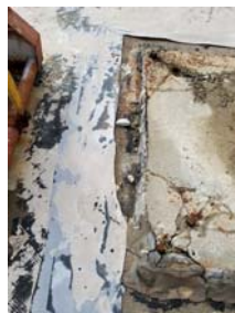
HMS-M17224-27A Mastic on Pad By Gear Device
