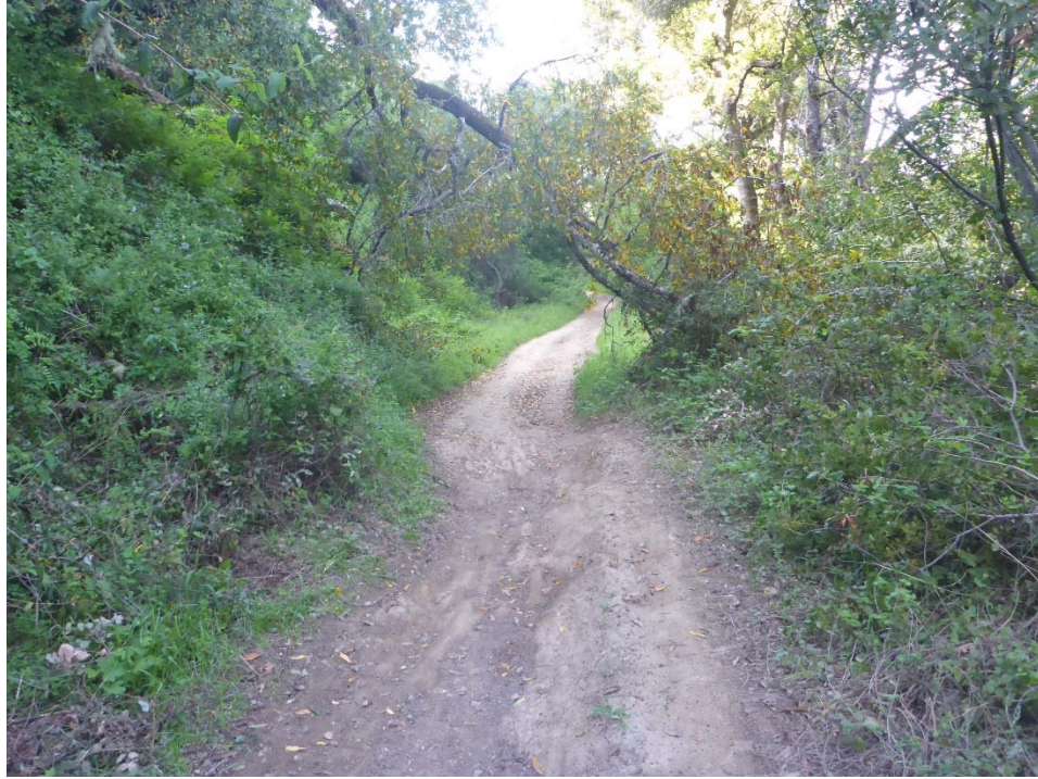
Photo 5. Representative photograph of access road within study area, showing minor rills from sheet flow after heavy rains.
