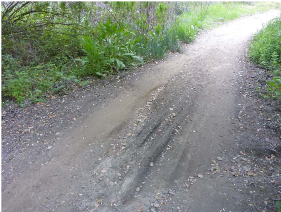
Photo 6. Representative photograph of access road within study area, showing minor rills from sheet flow after heavy rains.
