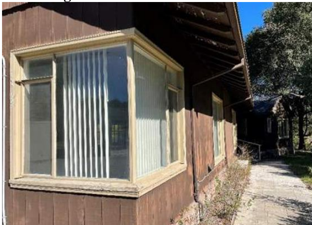
Figure 3. Steel Sash Window
