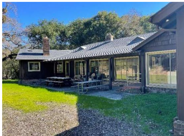
Figure 6. Partial View of The Rear North Side
