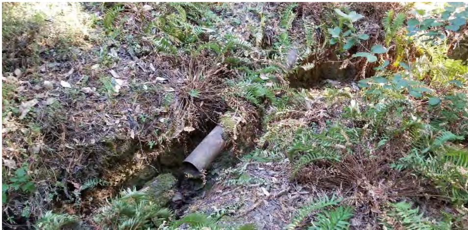
Photo 1: Looking downstream on diverted watercourse at skid trail crossing.
