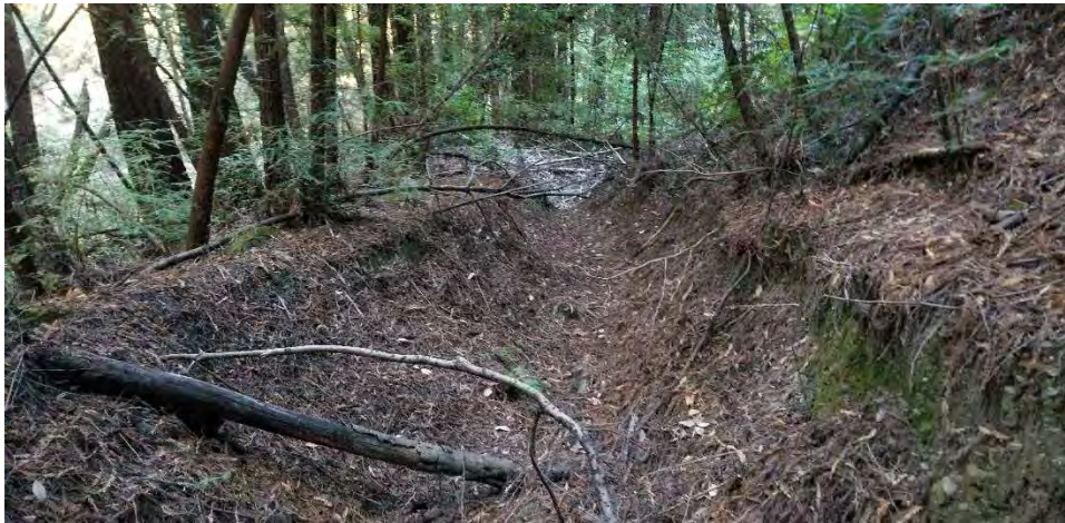
Photo 14: looking down the road at the eroded channel from diverted stream flow. This photo was taken along the lower portion of the gully where the incision is much greater. Note the heavy duff layer in the channel bottom.
