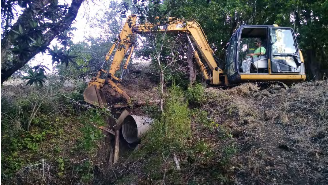
Figure 1 Existing old culvert
