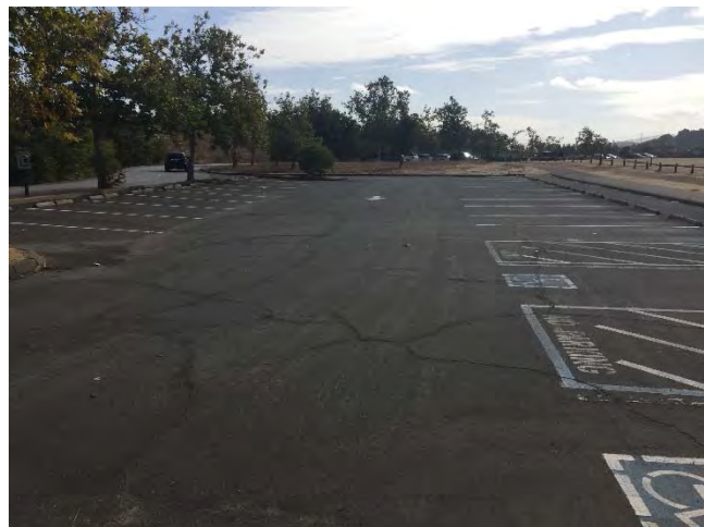
Lot 3 Facing South
