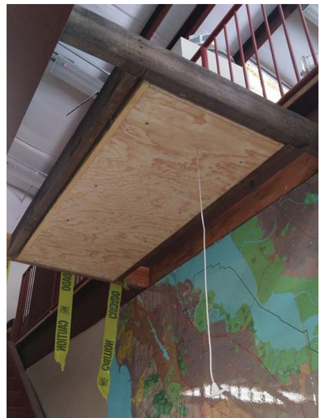
4. The ladder when closed sits flush with the framing and it is easy to operate.
