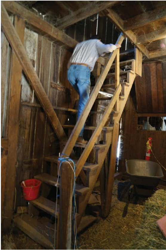
1. Stairs are steep with low headroom. Posts rest directly on soil.
