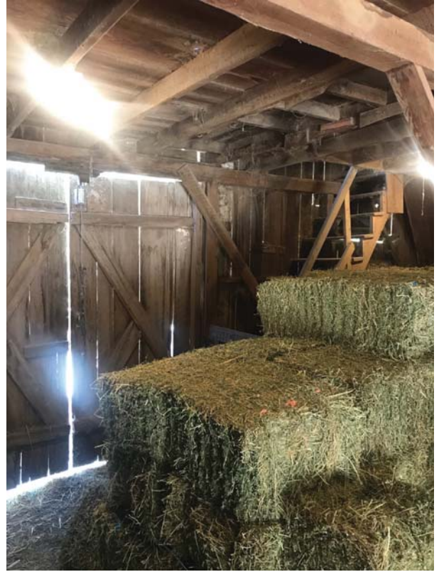
2 View of the stairs after a hay delivery.
