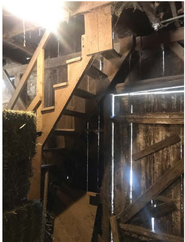
4 View behind the stairs.
