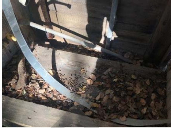
Photo 42. Woodrat A large amount of woodrat feces was observed in one location along the exterior of the structure.
