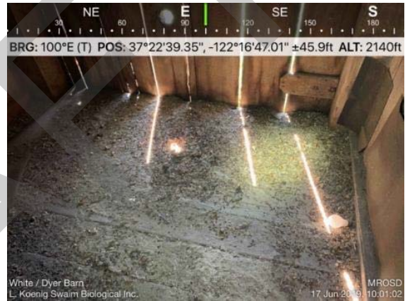
Photo 12. Rodent droppings and destroyed food caches observed within the barn.
