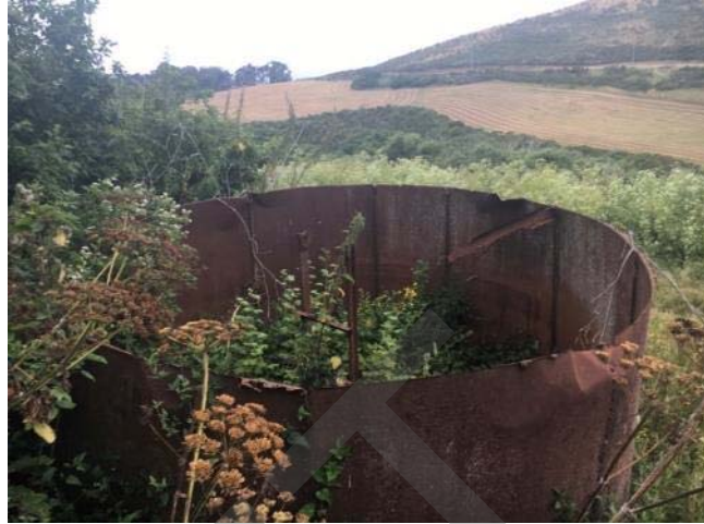
Photo 46. Area D – most tanks were single-walled without any small crevice space for roosting bats.
