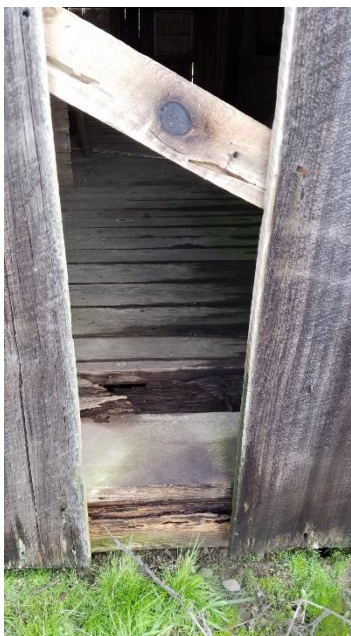
Photo 7. Deterioration at base of exterior wall
