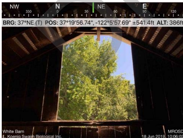
Photo 51. White Barn hayloft with crevice roost habitat between roof and rafters.
