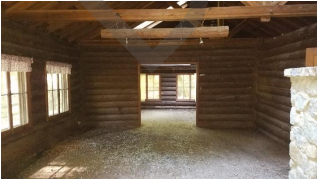
Photo 11. Interior view of main living room (note truss chords bearing on interior log walls and gaps evident between horizontal logs).
