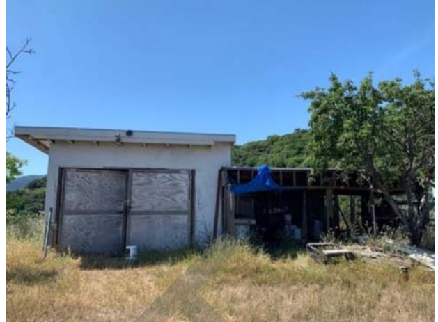
Photo 24. Structure C – shed west of Structure A.
