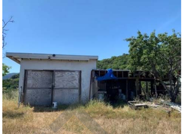
Photo 24. Structure C – shed west of Structure A.
