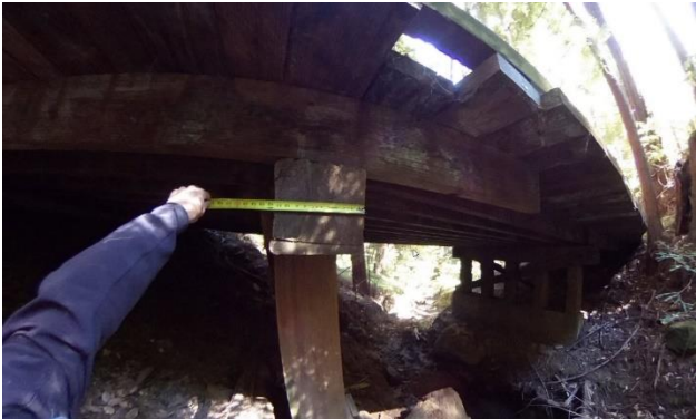
Photo 18. Timber bridge, second bridge to cross after 2nd gate.
