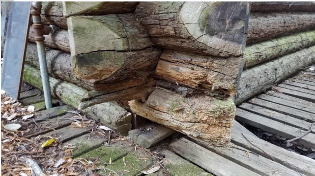
Photo 6. Close up of one of the areas of log wall corners showing signs of significant rot/decay
