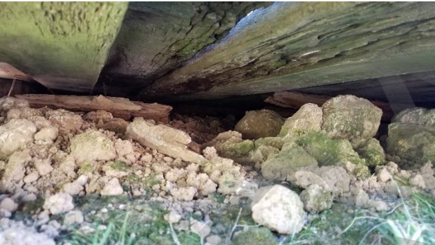
Photo 3. Existing condition at foundation
