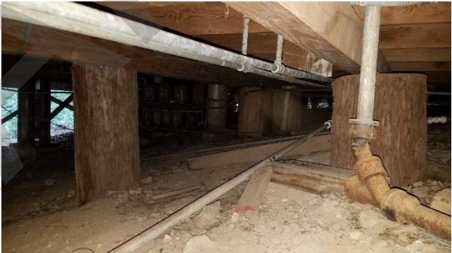
Photo 10. Ground floor framing and Interior log poles set directly into grade. Interior conditions are in fair condition.
