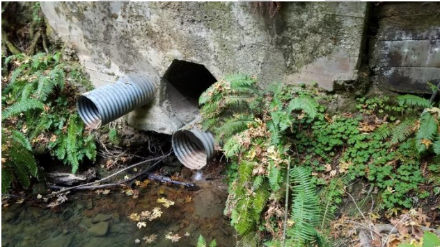
Photo 17. Earthen bridge, first bridge to cross after 1st gate, note portions of foundation appear to be undermined or scoured away from creek flow.
