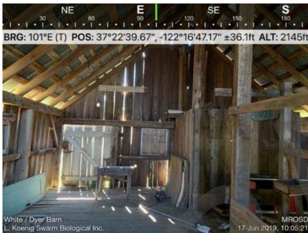
Photo 5. Interior of White Barn.
