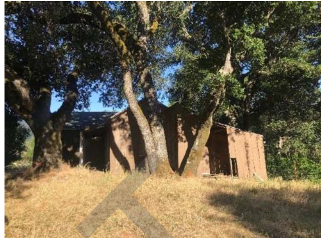
Photo 28. The housing structure is located beneath a canopy of coast live oaks (photo facing west).
