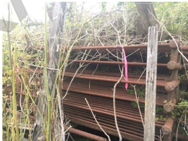
Photo 44. Area B – woodrat nest structure inside the series of iron grates. This structure sits over a concrete spring box filled with water.
