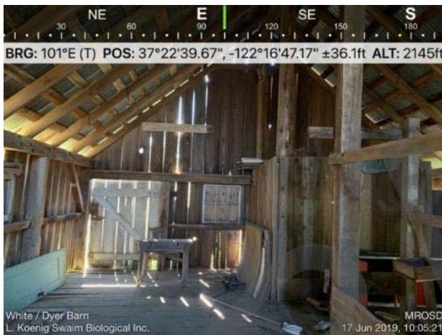
Photo 5. Interior of White Barn.
