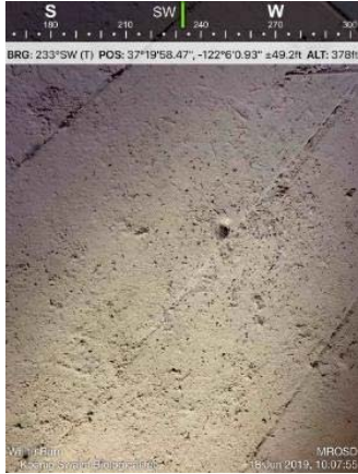
Photo 53. Bat guano on floorboards.
