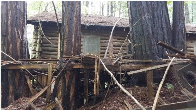
Photo 3. Partial rear (west) elevation of Structure, facing east (note collapsed deck framing)
