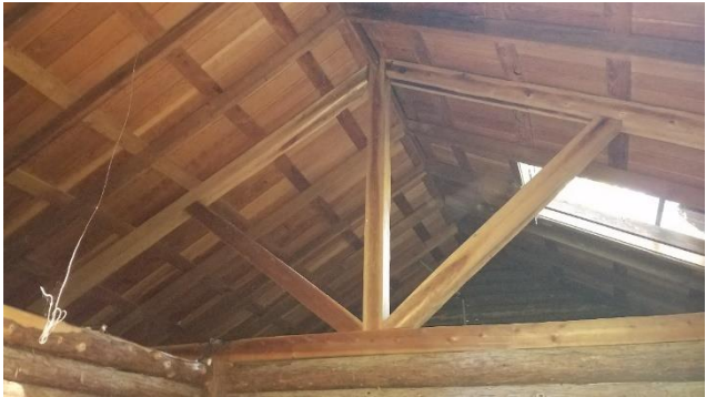
Photo 12. Interior view of roof framing, note gap at top chord showing evidence of load redistribution due to settlement of substructure.
