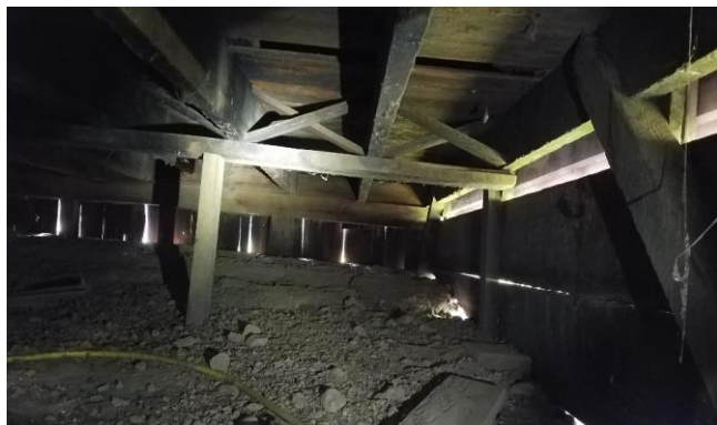
Photo 13. Crawlspace framing showing lack of concrete foundation, wood posts sitting directly on grade, and diagonal framing at perimeter wall
