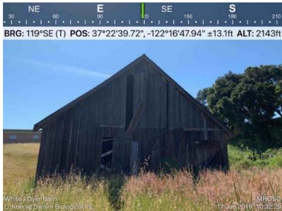
Photo 3. White Barn exterior missing wooden slats and entry points for bats.
