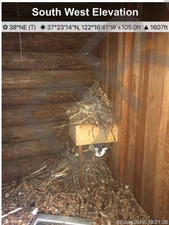
Photo 17. Woodrat nest on sink in Room A of redwood cabin.
