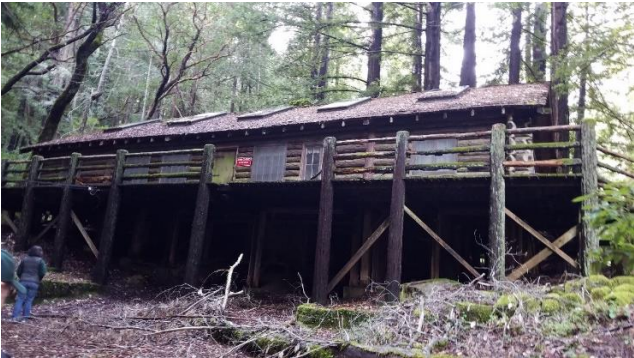
Photo 1. Front (east elevation) of structure, facing west (note missing guardrails)
