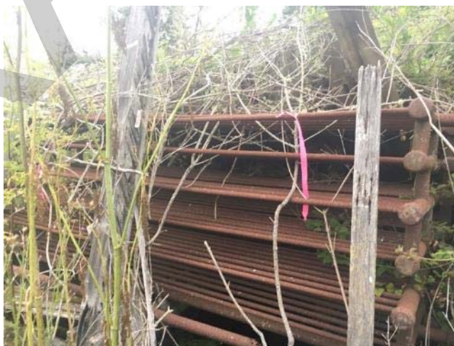
Photo 44. Area B – woodrat nest structure inside the series of iron grates. This structure sits over a concrete spring box filled with water.
