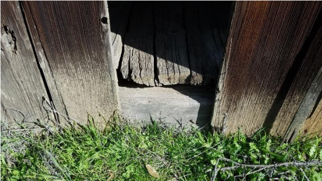
Photo 6. Deterioration at floor sheathing
