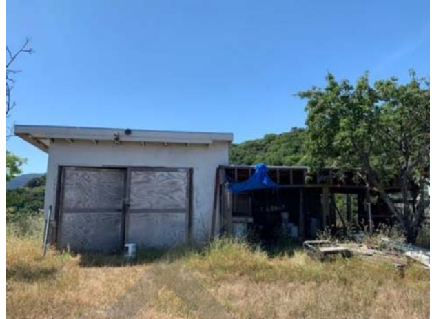
Photo 24. Structure C – shed west of Structure A.
