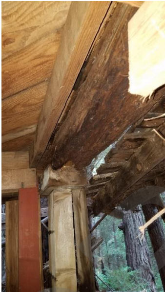
Photo 9. Area where dry rot/deterioration of base of log wall at corner of grid line D-1 was observed. This is likely a substantial contributor to the settlement observed in this area of the building.
