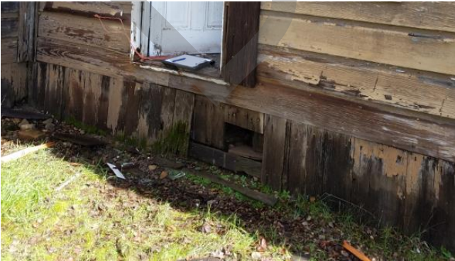
Photo 11. Moisture damage at exterior wall
