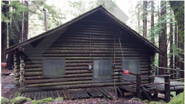
Photo 4. South wall elevation (note collapsed deck framing)
