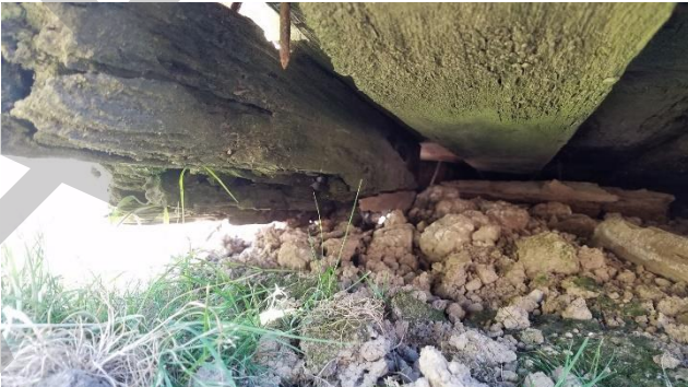
Photo 4. Existing condition at foundation
