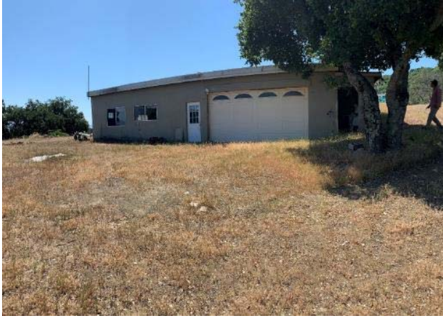
Photo 23. Structure B – north-side view.
