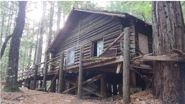
Photo 2. North elevation of structure, facing southeast (note collapsed deck area, failed railings and log wall displaced out of plane, observable by bend in conduit)
