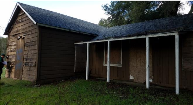
Photo 1. South elevation, showing shed roof support by posts
