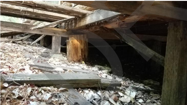
Photo 5. Log pole at south elevation (note severe rot and soil in contact)
