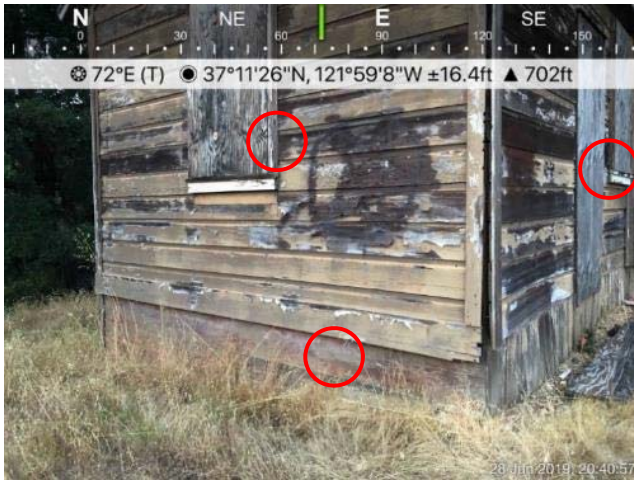
Photo 35. Bats observed emerging from wooden slats (circled in red) on west side of the house.
