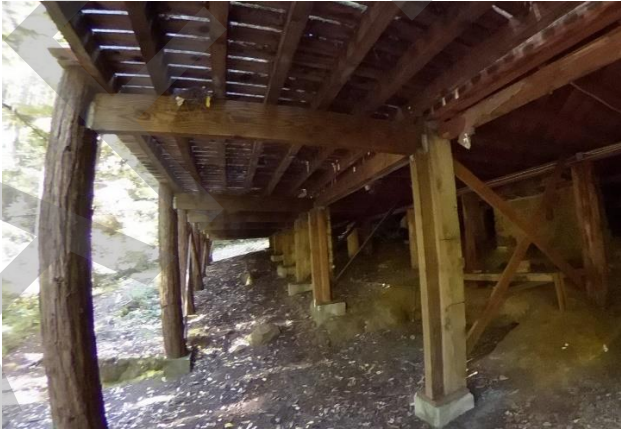
Photo 16. View of underside of deck and crawl space framing at east side of building (note concrete footings, fasteners and modern preservative treated lumber which shows that framing is not original).
