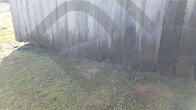
Photo 5. Deterioration of exterior siding
