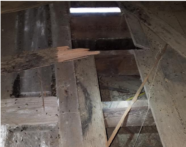
Photo 7. Missing wood planking at interior floor
