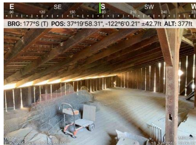
Photo 52. Interior of hayloft with wooden slat openings
