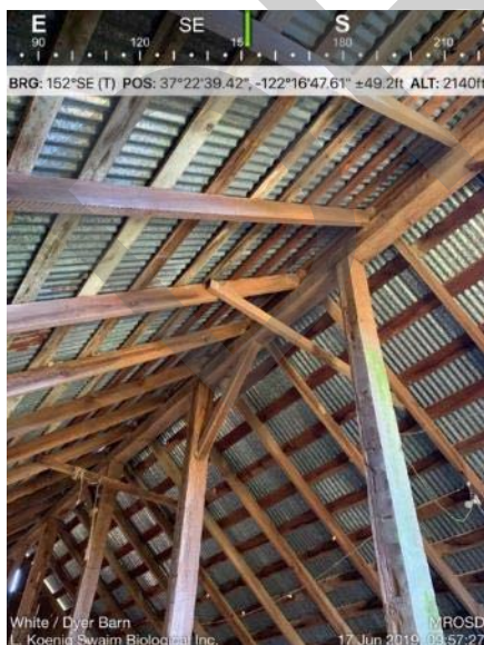
Photo 7. Corrugated roof slats and rafters provide suitable bat roosting habitat.
