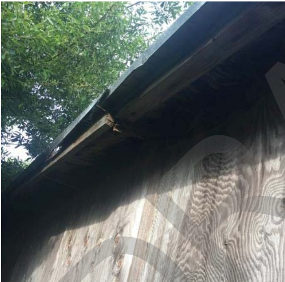
Photo 47. Area E – additional openings and interstitial spaces underneath the roofline.
