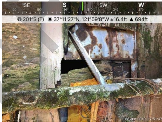
Photo 32. Hole on wall that could provide bat access.
