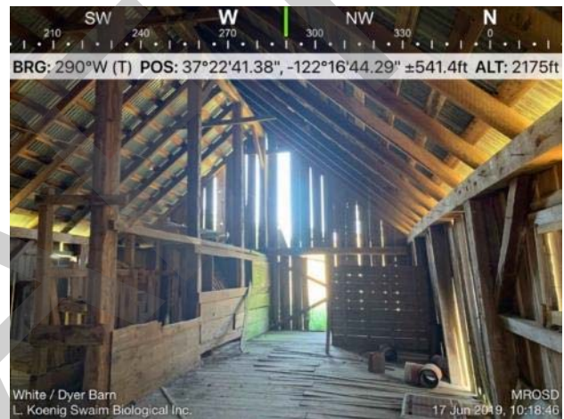
Photo 6. Interior of White Barn.
