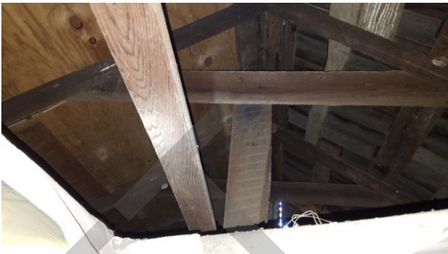
Photo 8. Hole in ceiling exposing collar ties, rafters, and 1x planking at roof
