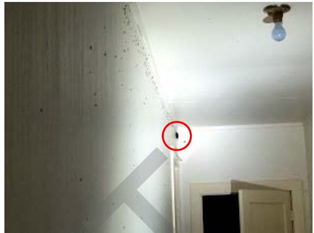
Photo 36. Bat urine staining and guano on wall; Myotis sp. (circled in red) observed roosting.
