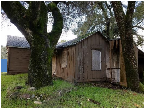
Photo 2. East elevation – dilapidated shed shown on the right
