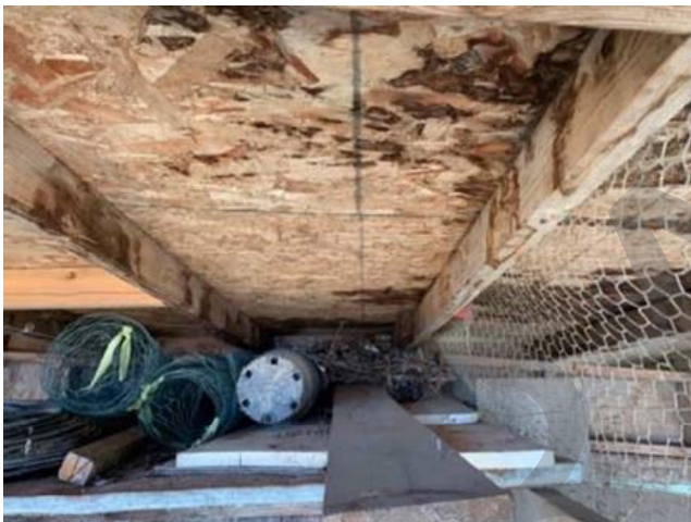
Photo 25. Possible woodrat midden on shelf in Structure C.
