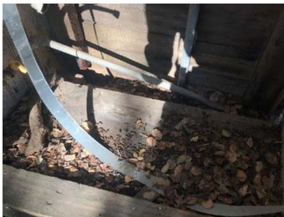
Photo 42. Woodrat A large amount of woodrat feces was observed in one location along the exterior of the structure.
