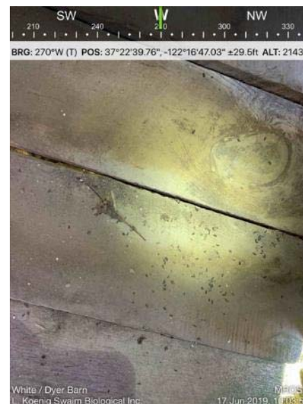
Photo 8. Bat guano present on the floor.
