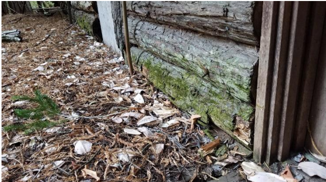
Photo 7. Area of base of log wall showing rot/decay (note buildup of debris on porch)
