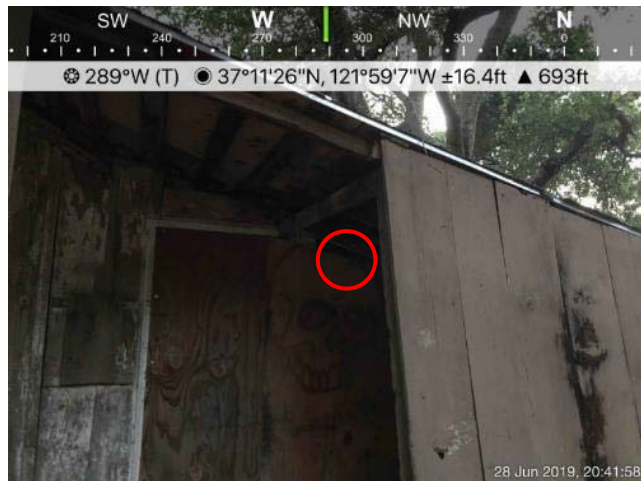
Photo 34. Bats observed emerging from hole in wall (circled in red) on east side of the house.
