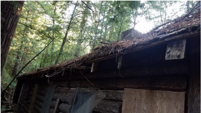
Photo 8. Location where significant buildup of leaves and debris have accumulated on the roof
