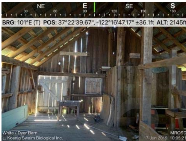
Photo 5. Interior of White Barn.
