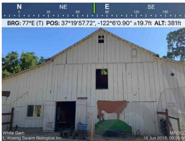
Photo 49. White Barn exterior showing hayloft doors and open access points.
