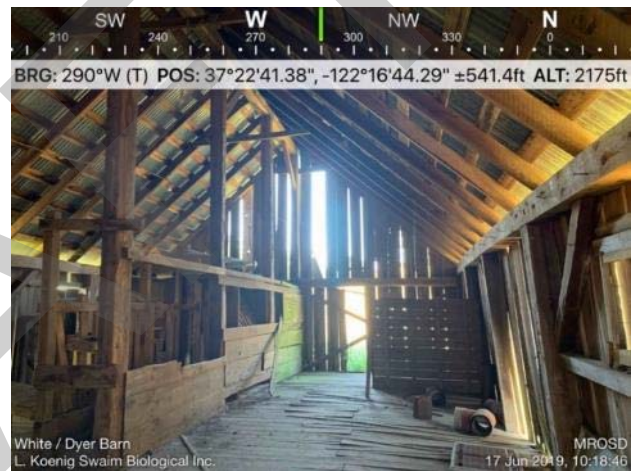
Photo 6. Interior of White Barn.
