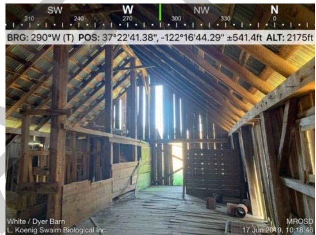
Photo 6. Interior of White Barn.
