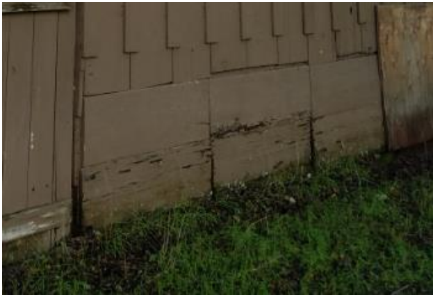
Photo 12. Moisture damage at exterior wall
