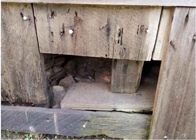
Photo 6. Missing siding on exterior wall, and lack of concrete foundation below bearing wall
