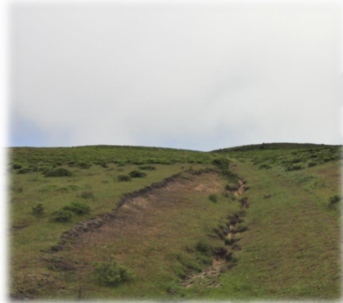
Figure-8: Gully/rutting activity along an insloped road just south of the farmstead. Large gully caused by surface water flow during winter storm events. Road should be re-graded and water diversion points installed to relieve surface flow to protect the integrity of the road.
