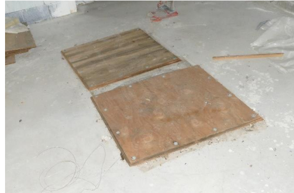
Figure 83. Plywood covering openings in floor.
