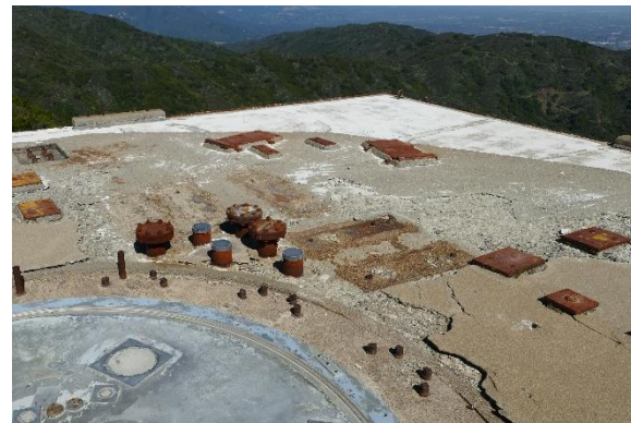
Figure 20. Steel plates, pipes, conduit, and other penetrations at the top of the concrete pedestal.
