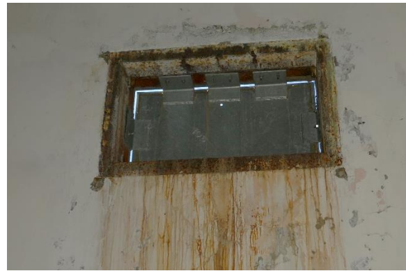
Figure 64. Water and corrosion staining below wall penetration.
