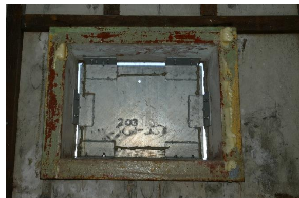
Figure 16. Interior of similar opening in concrete wall with gap around steel plate perimeter.
