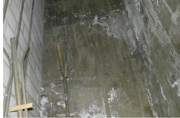
Figure 58. Efflorescence stains in utility shaft at southeast building corner, facing east.
