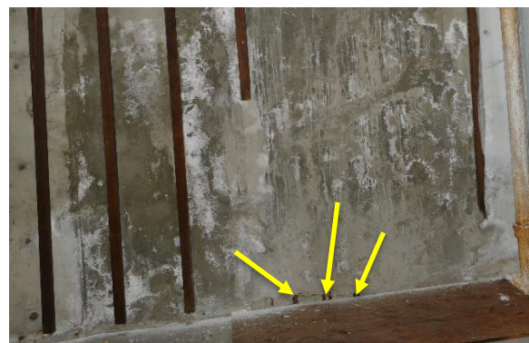
Figure 62. Exposed reinforcing steel observed along the base of the wall (arrows).
