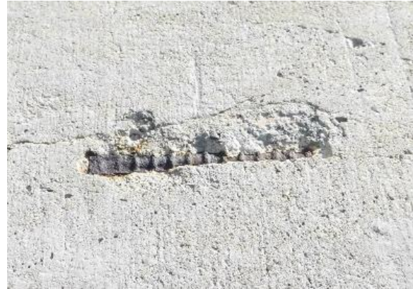
Figure 40. Reinforcing steel with little to no cover.
