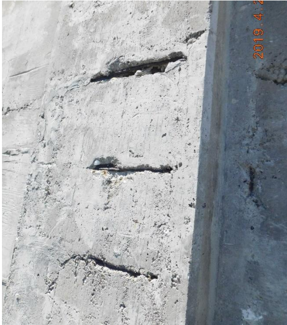
Figure 47. Concrete spalling on face of pilaster due to inadequate concrete cover.
