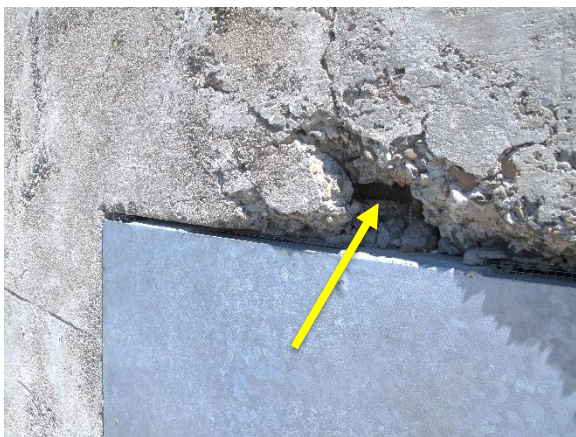
Figure 65. Concrete spalling and exposed reinforcing steel (arrow) adjacent to infilled window opening.
