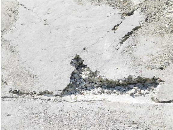
Figure 43. Poorly consolidated concrete above the horizontal construction joint above the floor slab with a smooth patch area above.
