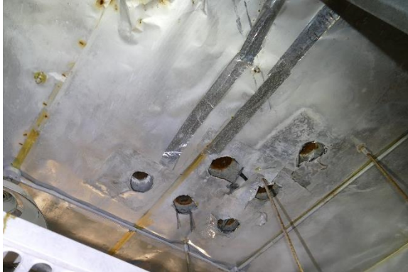
Figure 74. Aluminum sheets installed beneath the roof slab are noted as radar shielding in the construction drawings.
