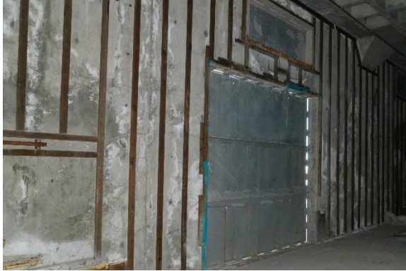
Figure 57. Efflorescence stains at interior of concrete walls.
