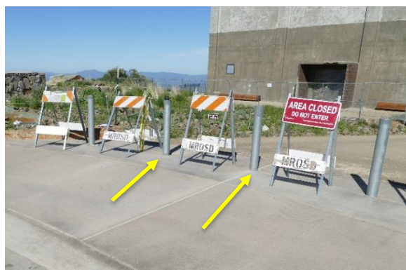
Figure 88. Bollards along the sidewalk. Arrows indicate the two removable bollards.
