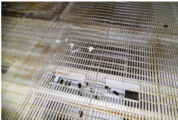
Figure 84. Rectangular holes in the mezzanine floor grating are large enough to accidentally step through.
