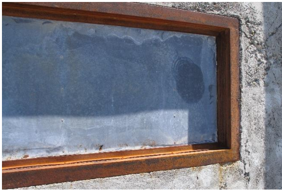
Figure 63. Galvanized steel plate with light oxidation and corroded steel frame.
