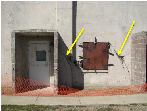
Figure 45. Cracks visible at east elevation (arrows). (Photo taken in 2013 by WJE)
