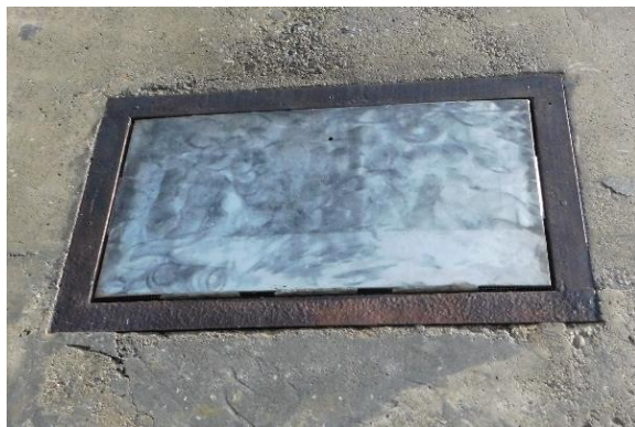
Figure 15. Typical opening in concrete wall, closed with steel plate.
