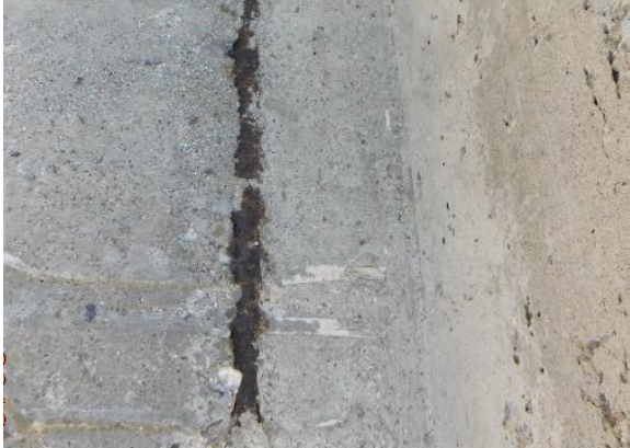
Figure 39. Corroded reinforcing steel with minimal concrete cover.
