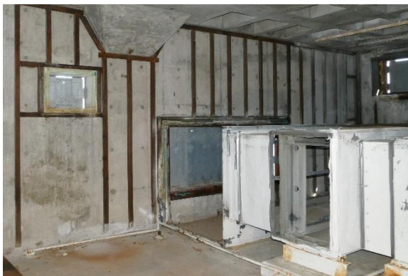
Figure 35. The building interior has remaining wood-framed partitions, furring and some abandoned HVAC equipment.
