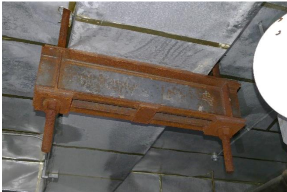
Figure 76. Surface corrosion on steel beam clamp.
