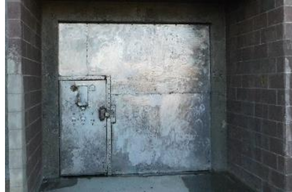
Figure 87. The west door was originally a double-leaf door, but appears to have been modified and has only a small access door in a larger metal plate.
