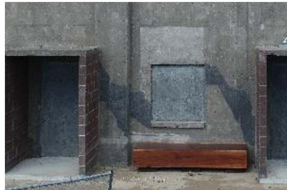
Figure 46. Repaired cracks and infilled openings at east elevation.
