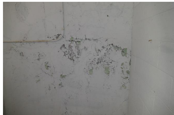
Figure 60. Peeling paint on the inside face of the exterior wall.
