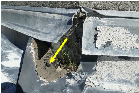
Figure 69. Damaged counterflashing at concrete pedestal showing single-ply membrane flashing (black sheet, damaged), fluid-applied coating (white), and original built-up flashing (black residue adhered to interior surface of single-ply flashing, arrow).
