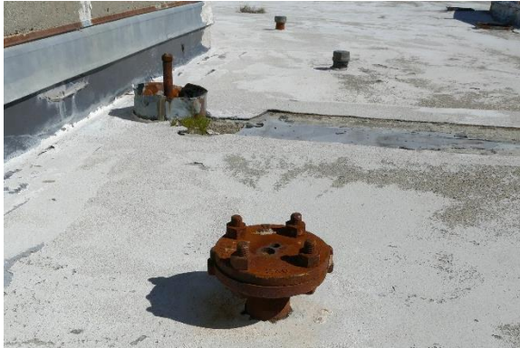
Figure 21. Various pipe penetrations, conduit in a pitch-pocket, and visible sealant repairs at the expansion joint. Photo facing north.
