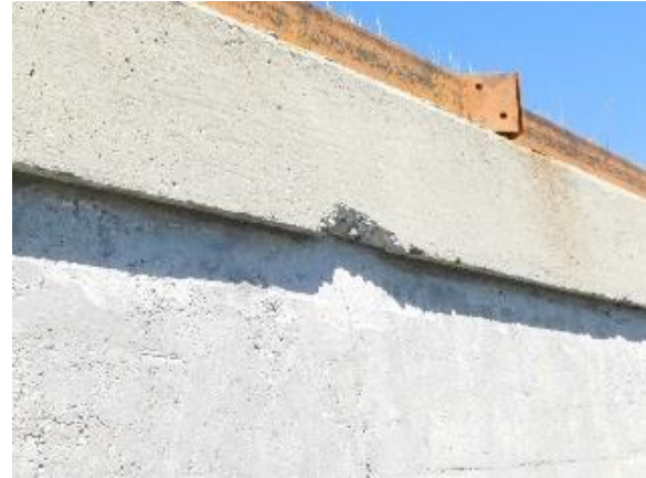
Figure 54. Small concrete spall along the bottom edge of perimeter roof edge beam.
