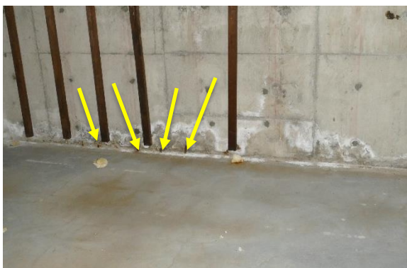
Figure 61. Exposed reinforcing steel observed along the base of the wall (arrows).
