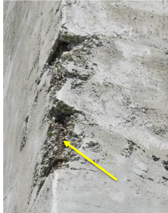
Figure 50. Poorly consolidated concrete on the sides and corner of the pilaster. Note exposure of reinforcement steel (arrow).
