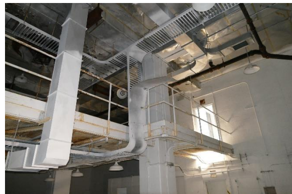
Figure 36. Steel-framed mezzanine at the fifth floor.
