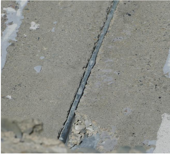
Figure 30. Wearing slab expansion joint formed from folded copper sheet that was originally covered by sealant. Note that the other three joints in the slab were concealed by more modern repair sealant.
