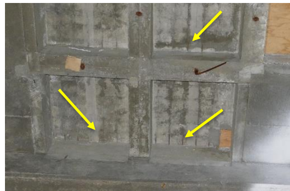
Figure 81. Corrosion staining of reinforcing steel at the soffit of the fifth floor (arrows)
