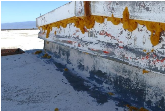
Figure 67. Single-ply membrane flashing (black), spray foam (yellow), and fluid-applied coating (white) at roof equipment hatch.
