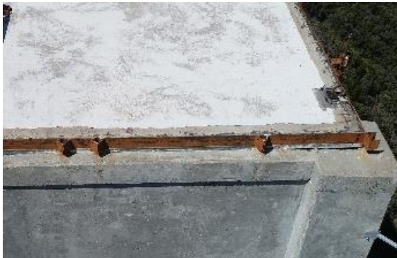
Figure 25. Perimeter brackets for supporting guardrail.
