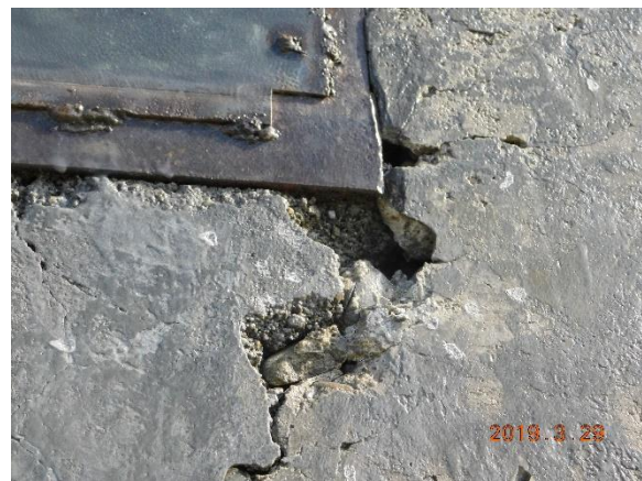
Figure 66. Voids in concrete due to poor consolidation adjacent to window opening.
