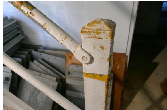
Figure 77. Surface corrosion on metal stair handrail.
