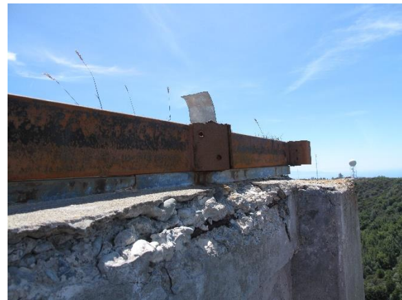
Figure 52. Concrete spalling and exposed reinforcing along the perimeter roof edge beam.
