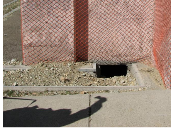
Figure 34. Utility trench beneath the south end of the east elevation in 2013, prior to construction of the site pathway. Photo facing west.
