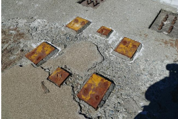
Figure 70. Concrete spalling and corroded steel plates on the top surface of the concrete pedestal.
