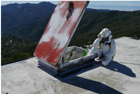
Figure 23. Roof hatch near east edge of roof, facing southeast.
