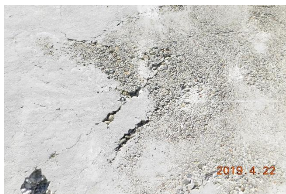
Figure 38. Concrete with a rough surface and areas of poor consolidation.
