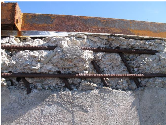
Figure 51. Concrete spalling and exposed reinforcing along the perimeter roof edge beam.
