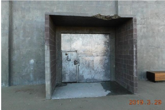
Figure 17. Covered exterior entryway around main entry door on west elevation. Note the spall at the edge of the roof slab.
