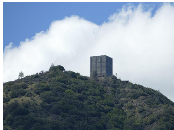
Figure 4. Photo of the radar tower, facing west.
