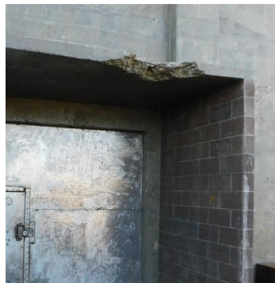
Figure 56. Spalling of concrete slab at top of roof of wind screen.
