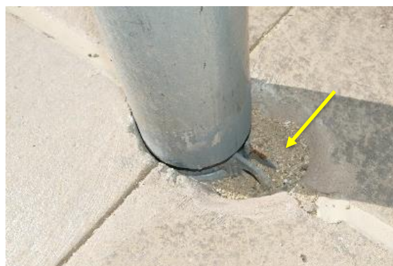
Figure 89. Base of removable bollard. Note sand in the recess adjacent to the bollard sleeve (arrow).
