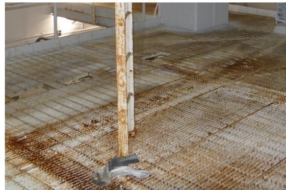
Figure 85. Surface corrosion at mezzanine floor grating below concrete pedestal at roof above.
