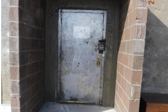
Figure 86. Steel door at south of east wall.
