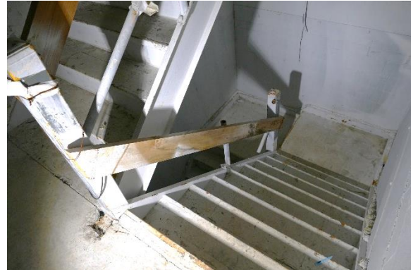
Figure 79. Partially missing handrail with temporary wood railing.
