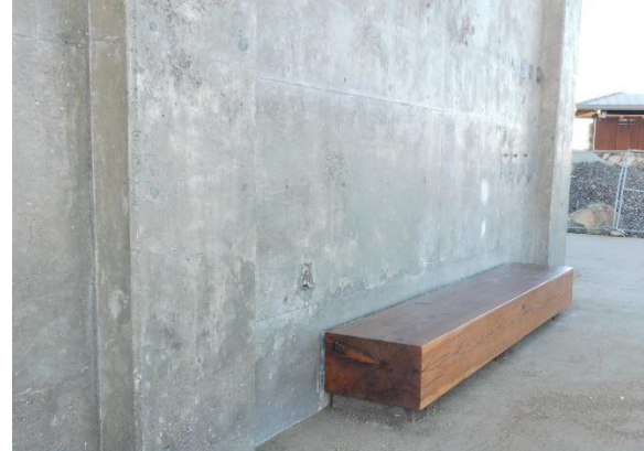
Figure 11. Wood bench installed close to exterior wall.
