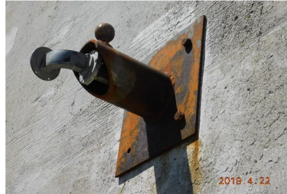
Figure 18. Steel fixture attached to concrete wall.
