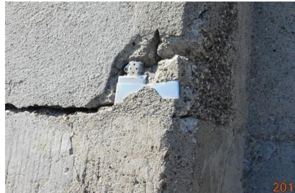
Figure 42. Cigarette lighter embedded in the concrete wall on the south elevation.
