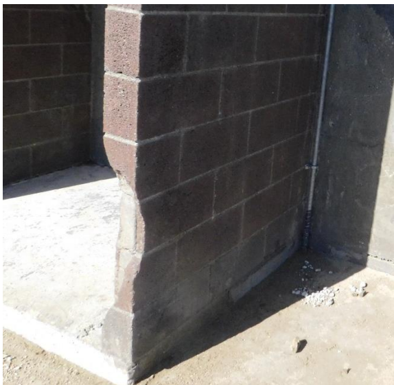
Figure 55. Spalling of concrete block wall of wind screen
