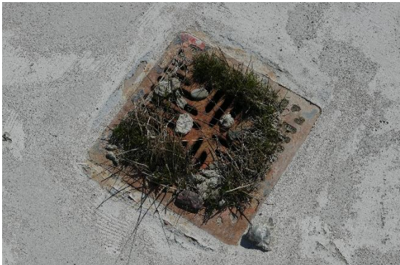
Figure 32. One of four area drains with plants growing out of the drain.
