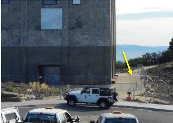
Figure 10. Pathway (arrow) from parking area to east peak lookout adjacent to the building.
