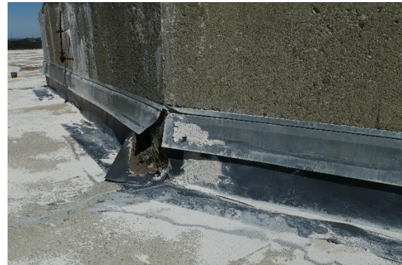
Figure 28. Counterflashing at concrete pedestal. Note the single-ply membrane flashing that was later added, and has failed.
