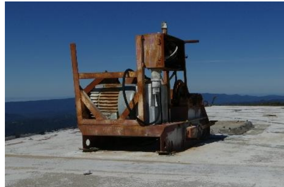
Figure 24. Rooftop equipment, facing southwest.
