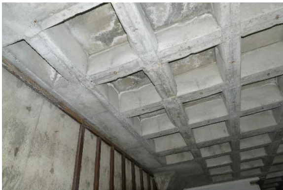
Figure 59. Efflorescence visible on the underside of the third floor slab where water leaks into the building and through the slab.
