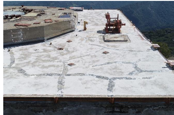
Figure 68. White traffic coating on main roof, facing east. Note the darker stripes where underlying cracks were treated.
