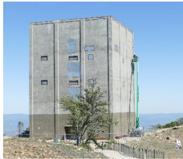
Figure 2. Recent exterior view of the radar tower facing east.
