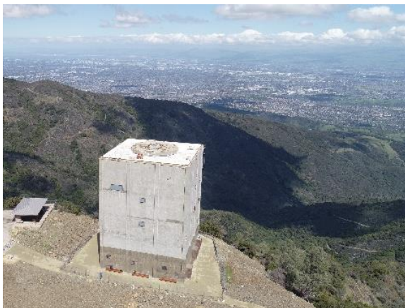
Figure 3. Aerial photo of the radar tower, facing north.
