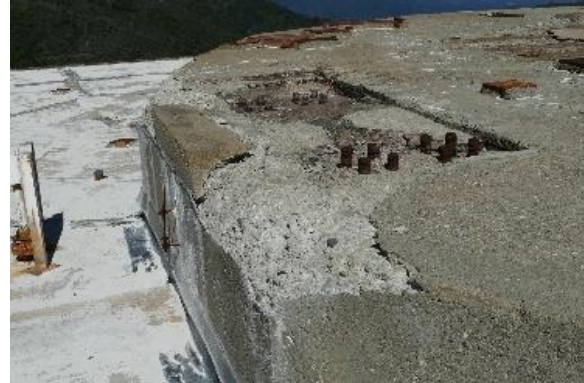
Figure 71. Concrete spalling along the edge of the concrete pedestal.
