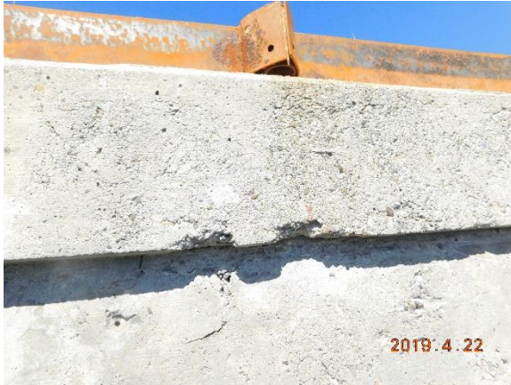
Figure 53. Small concrete spalls along the bottom edge of perimeter roof edge beam.
