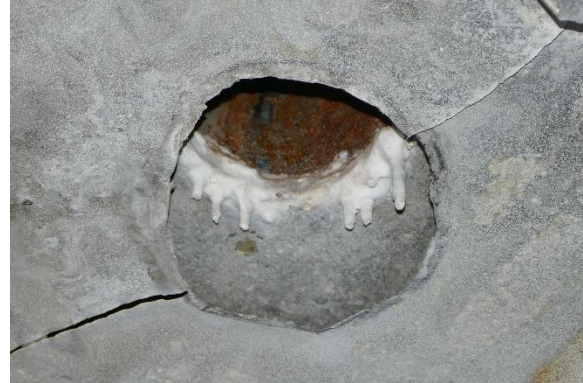
Figure 75. Efflorescence deposits around penetration in concrete roof slab, with aluminum sheets in foreground.
