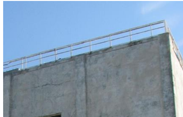
Figure 26. Apparently metal guardrail that was present circa 2013.
