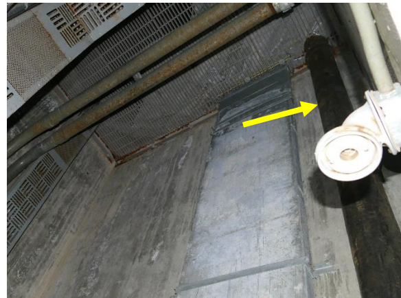
Figure 73. Cast iron drainage plumbing stack in utility shaft. Photo facing southeast.
