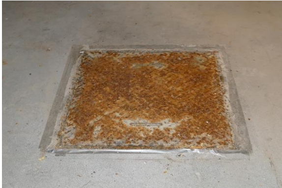
Figure 82. Corroded metal plate covering opening in floor.
