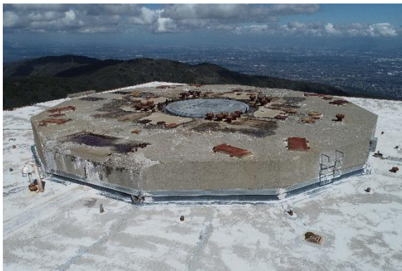
Figure 19. Concrete pedestal that once supported the radar antenna, facing northwest.
