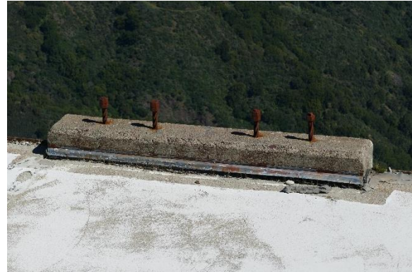
Figure 22. Curb with counterflashing at roof edge, facing north.
