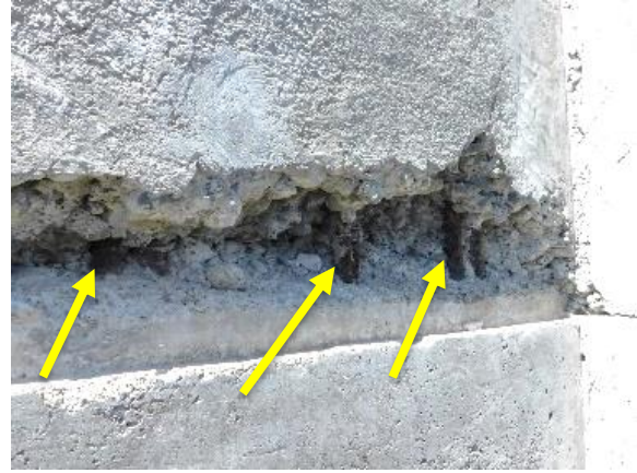
Figure 44. Poorly consolidated concrete above the horizontal construction joint above the floor slab revealing the joint key and reinforcing steel (arrows).
