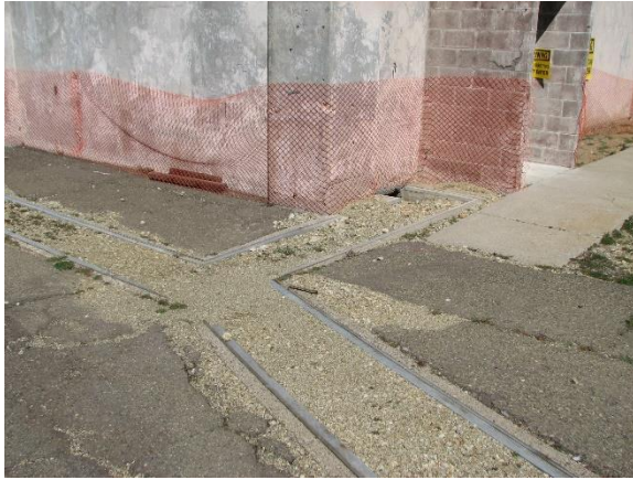
Figure 33. Utility trenches at the southeast corner of the Radar Tower in 2013. Photo facing northwest.
