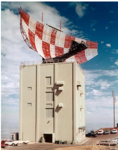
Figure 1. Historic photo of Mount Umunhum radar tower facing east. Photo courtesy of Midpeninsula Open Space District.
