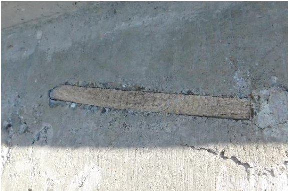
Figure 41. Piece of wood embedded in the concrete wall on the east elevation.
