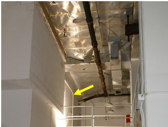
Figure 72. Cast iron drainage plumbing with widespread corrosion running into the utility shaft at the southeast corner (arrow). Photo facing south.
