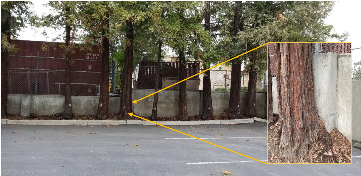
Figure 14: Trees 71-78 (left to right). Tree 73 is shown close up on the right and shows how the tree is growing against the concrete wall.
