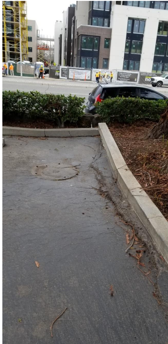
Figure 10: Curb damage seen caused by trees 35 and 36.
