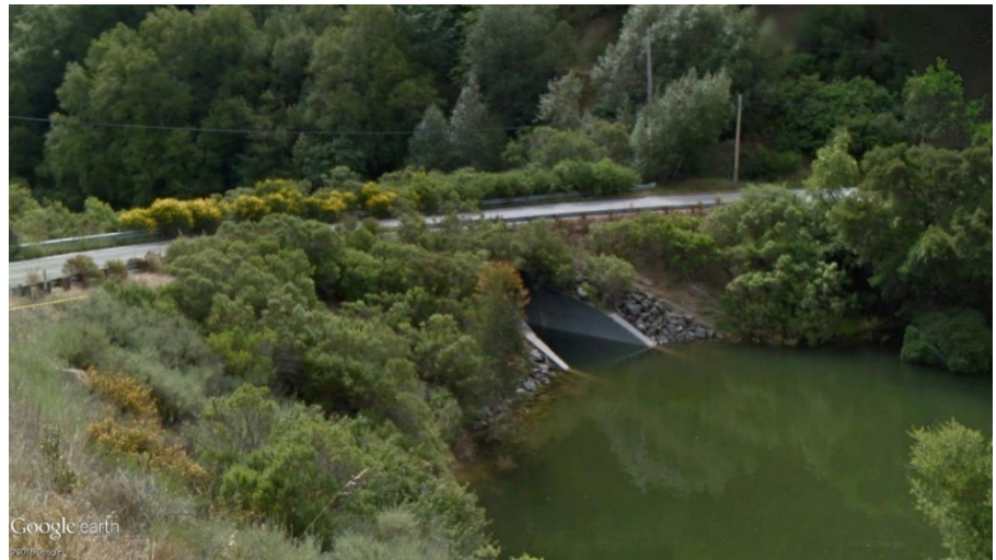
Type 3: Above large culvert at Limekiln Creek
