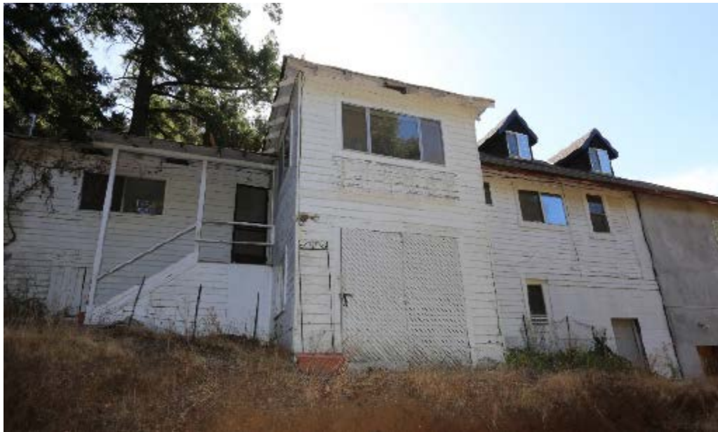
Lysons – Upper House Side View
