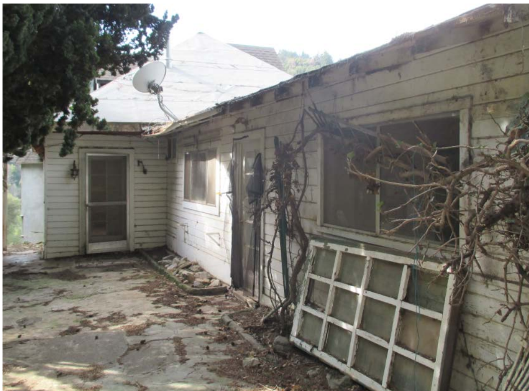
Lysons– Upper House Back Patio Area
