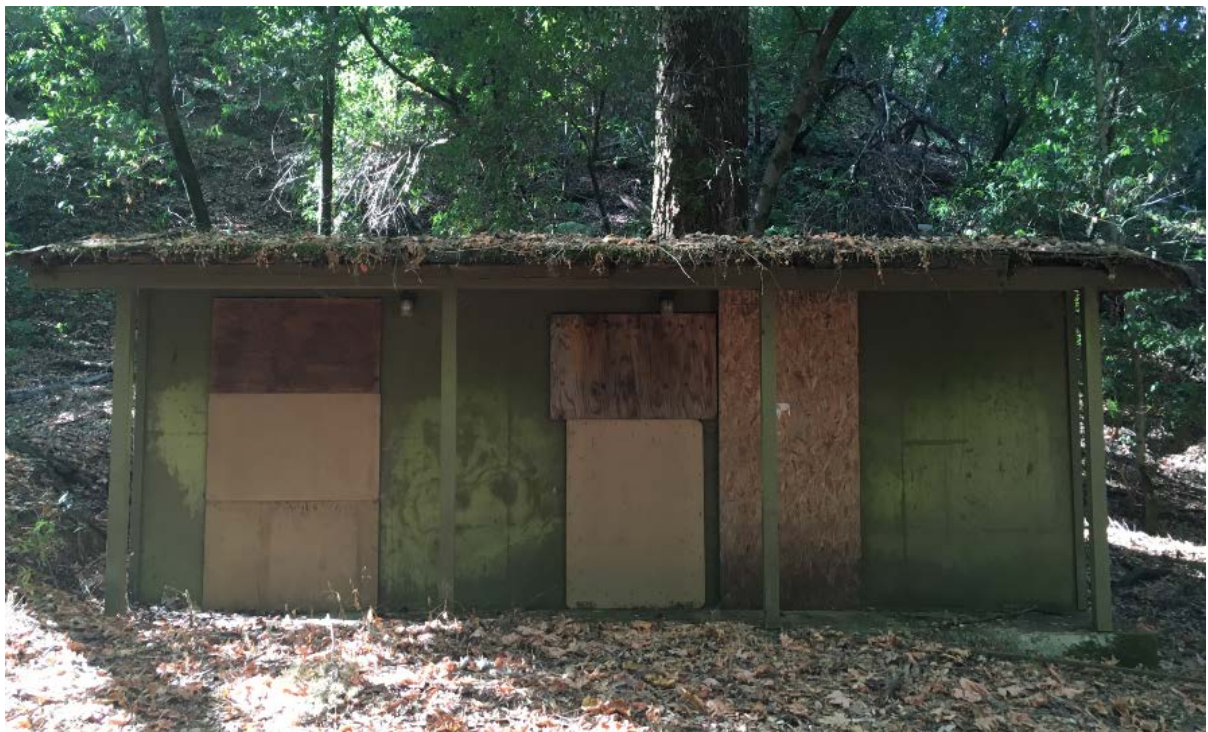
Stevens Canyon Ranch – Restroom Structure
