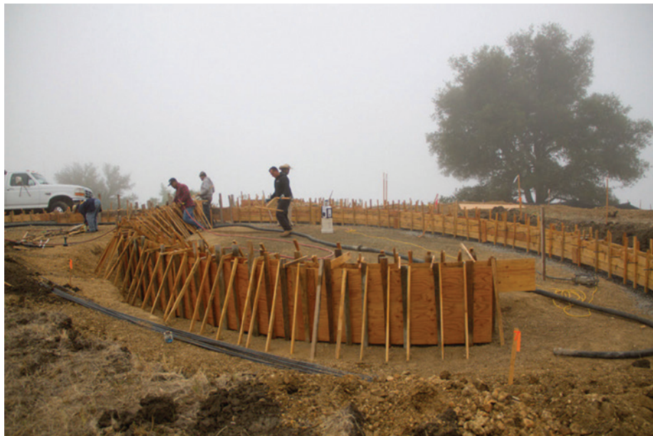
Mindego Gateway Construction, Russian Ridge Open Space Preserve by District Staff
