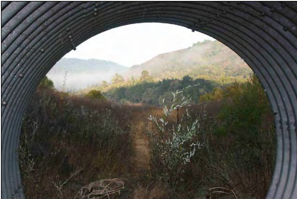
Figure A20: Culvert 3, west side, picture taken in July 2010.
