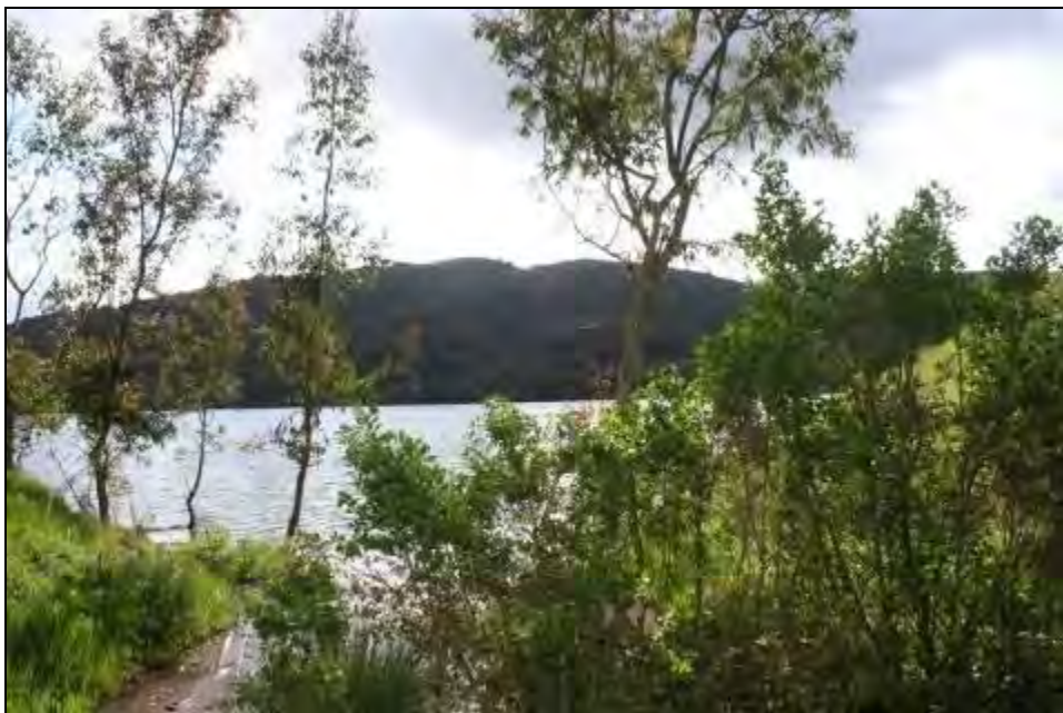
Figure A22: East view of Culvert 3 on east side leading into Lexington County Park and Reservoir.
