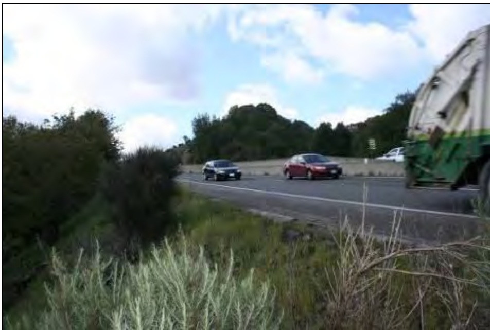
Figure A5: Standing at road where fence is down.
