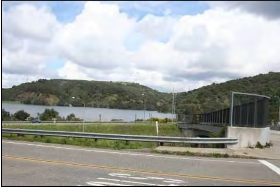
Figure A17: North side of Alma Bridge. Potential site for adding in additional lane for wildlife.
