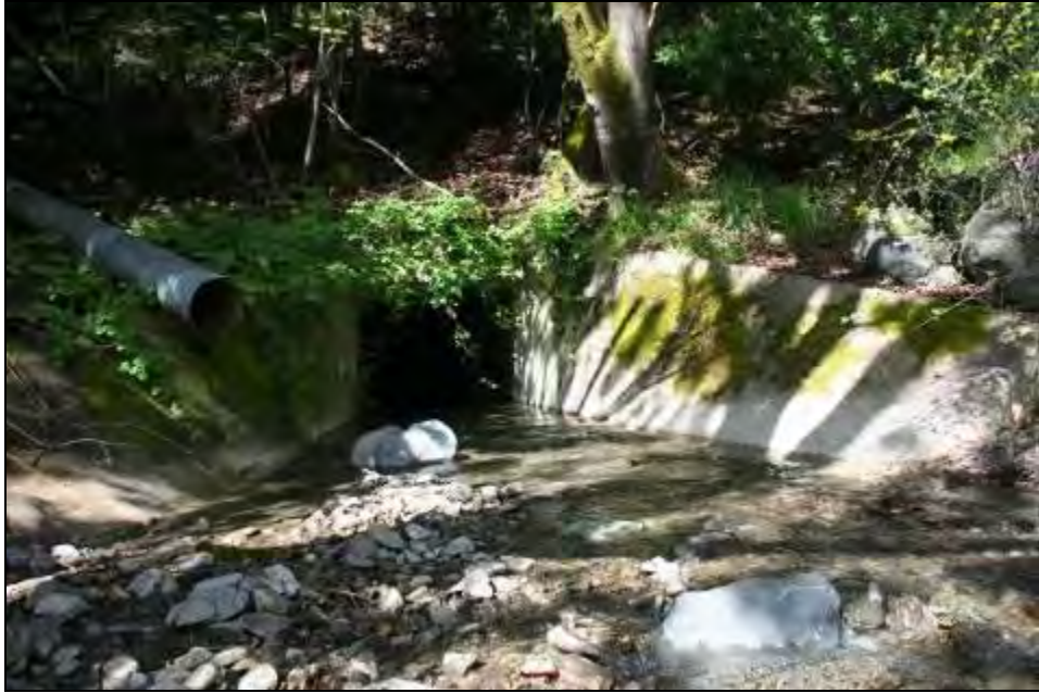
Figure A13: Culvert 2, east side, not visible through.
