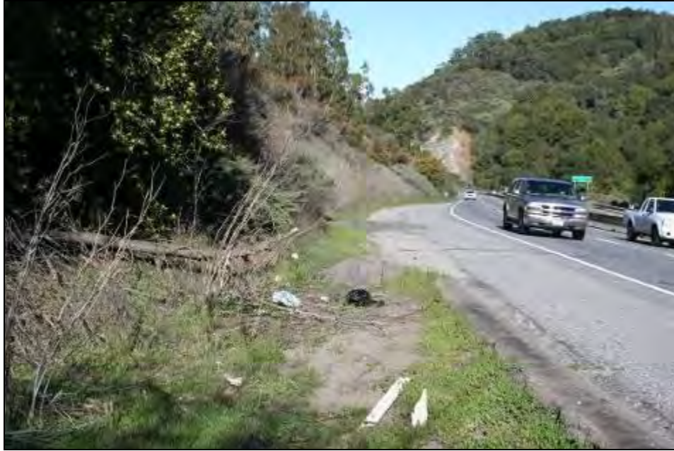
Figure A6: Site where Puma was hit at southbound Hwy 17 on 2-9-2011, northbound view.
