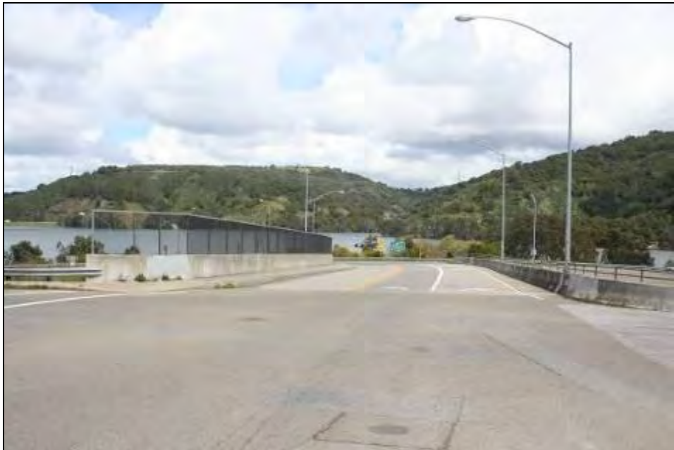
Figure A16: Alma Bridge, west side.
