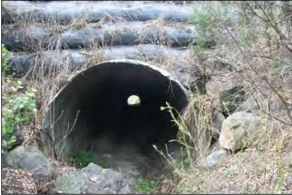
Figure A15: Culvert 3, east side at Lexington Reservoir.
