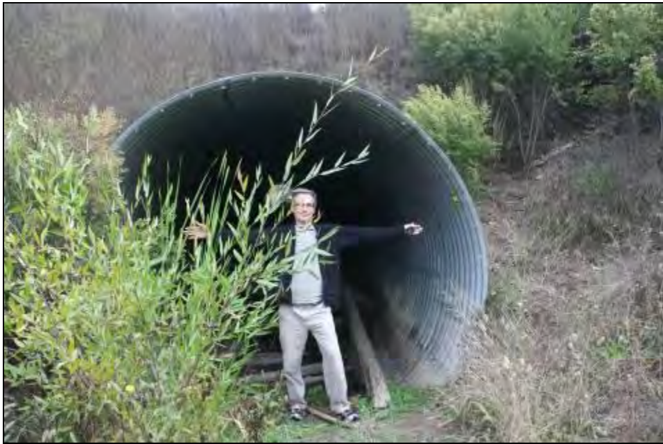
Figure A14: Culvert 3, west side, visible through.
