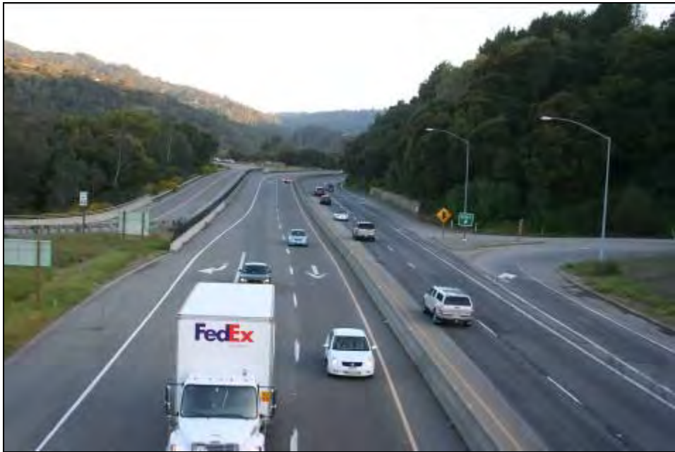
Figure A2: Concrete median in Highway 17, south view.
