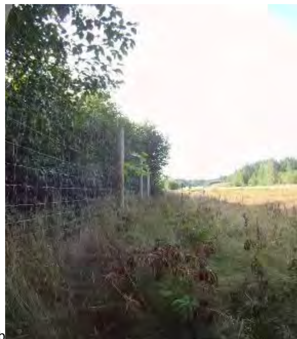
Figure 4 An eight-foot-tall fence-line in Canada. a) The fence is anchored to the bridge abutment, allowing wildlife to pass under the bridge, over a stream; b) The fence is continuous for many miles, preventing wildlife access to the highway.
