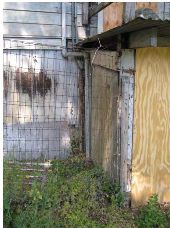
Image 9. Sewer lateral on south side of Cottage
