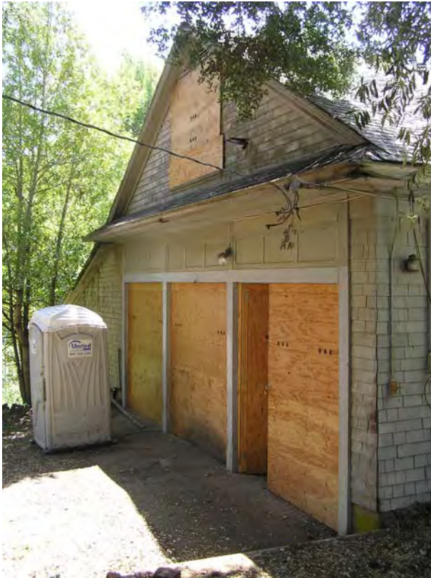
Image 70. Garage, north façade, view of the garage openings.
