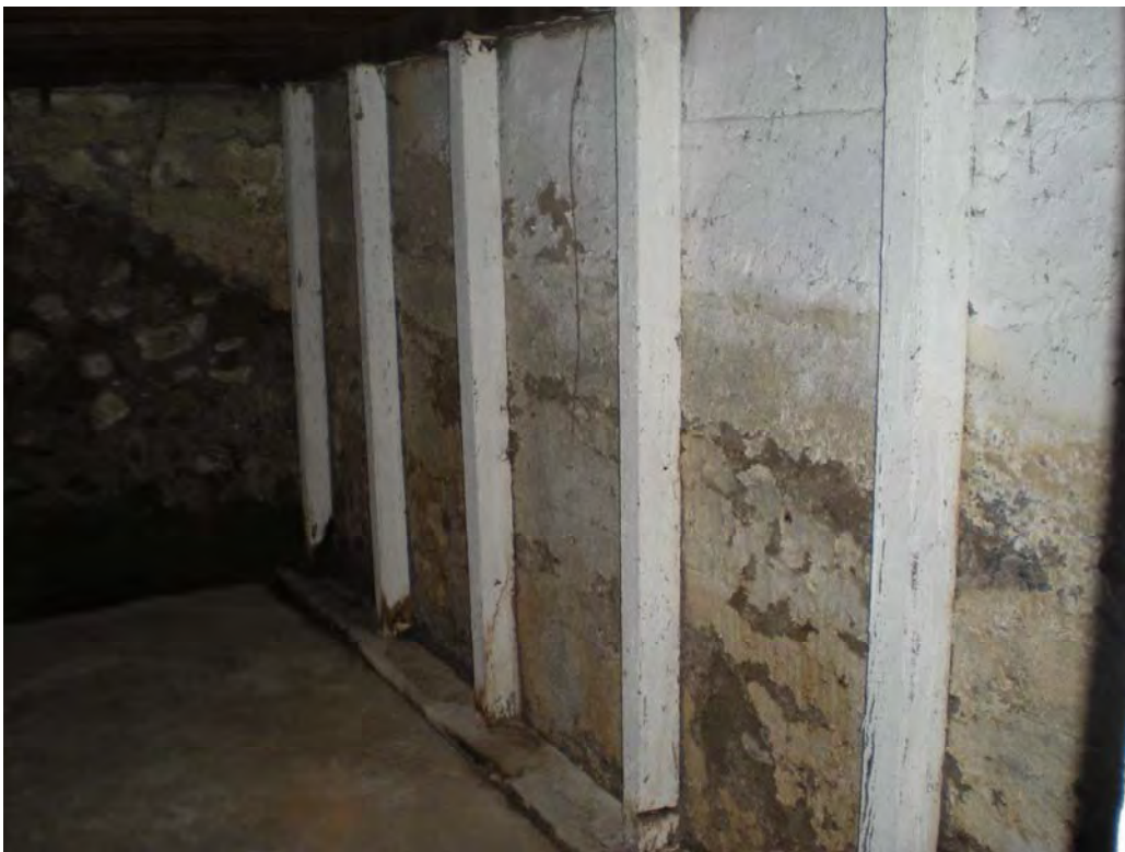
Image 35. Hawthorn House, Basement, Room A, north wall looking northwest.
