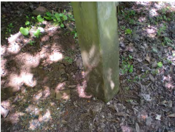
Image 83. Garage, east lean-to addition, post on grade.
