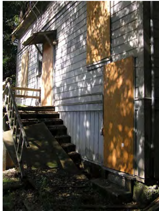
Image 106. Cottage, east entry stair.
