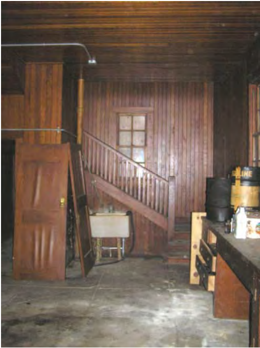
Image 75-76. Garage, stair to attic.
