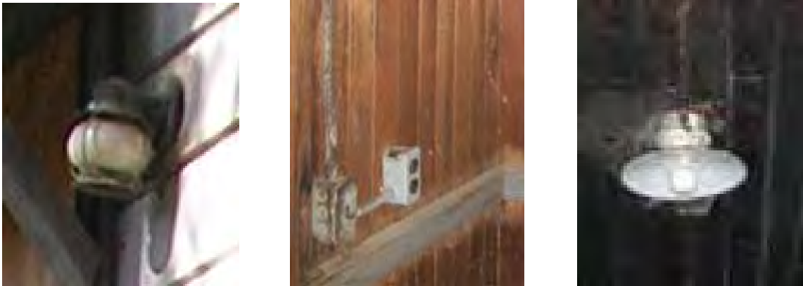
Image 117-119. Exterior Lantern; Surface Conduit & Receptacle; Cone Shade Fixture
