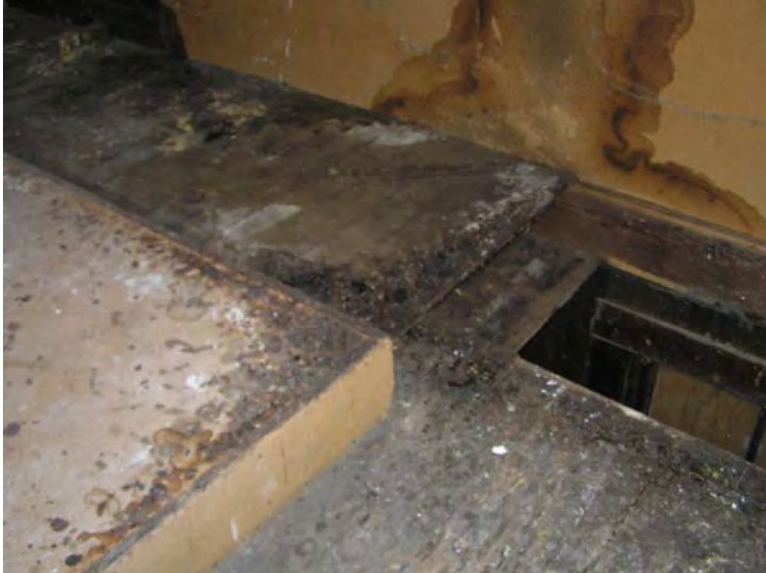
Image 109. Cottage, Attic floor at platform and ladder/stair opening.
