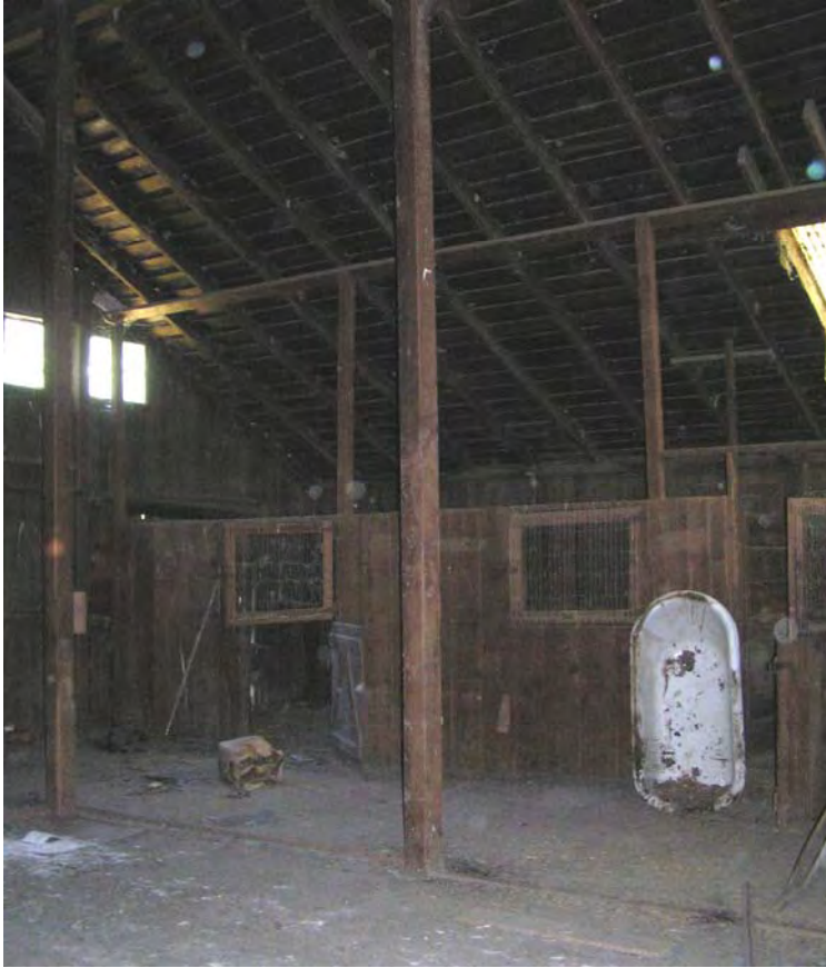
Image 123. Lower Barn, interior looking northeast.
