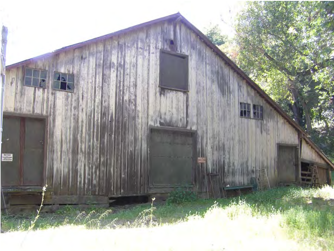
Image 120. Lower Barn, north façade.
