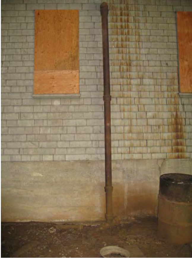
Image 10. Sewer Service at the east Garage façade under the east lean-to addition.
