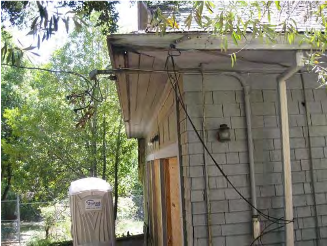
Image 98. Garage, electrical wires at exterior northwest corner.
