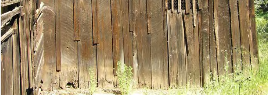
Image 125. Dry rot at base of walls.
