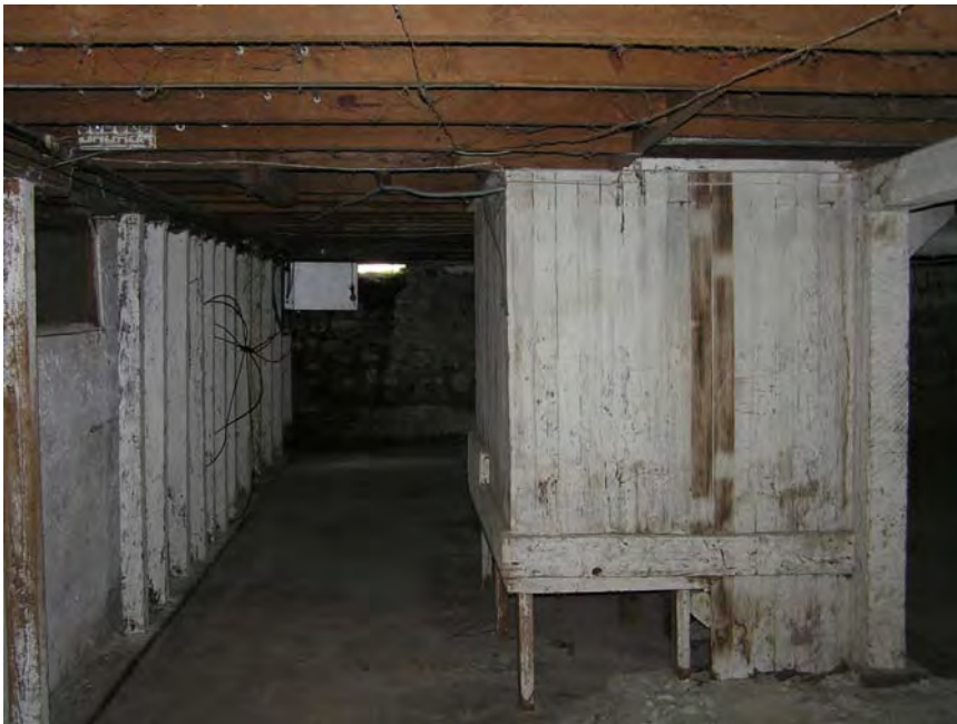
Image 21. Hawthorn House, Basement looking west, Stair 2 enclosure in the foreground.
