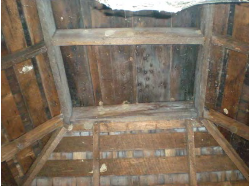
Image 114. Cottage, roof framing and sheathing as seen from the attic.
