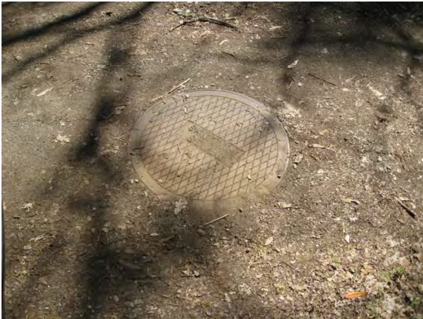
Image 11. West Bay Sanitation District sewer manhole at the pipeline, which serves the Portola Valley Ranch development south of the Hawthorns property.
