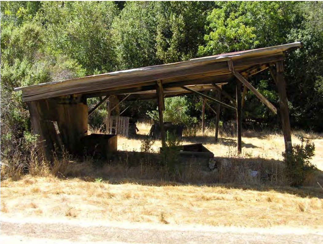
Image 135. Outbuildings, Horse Sheds, two of four.
