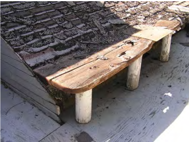
Image 80. West deck, severe deterioration at attic entry side walls and bench at eave.
