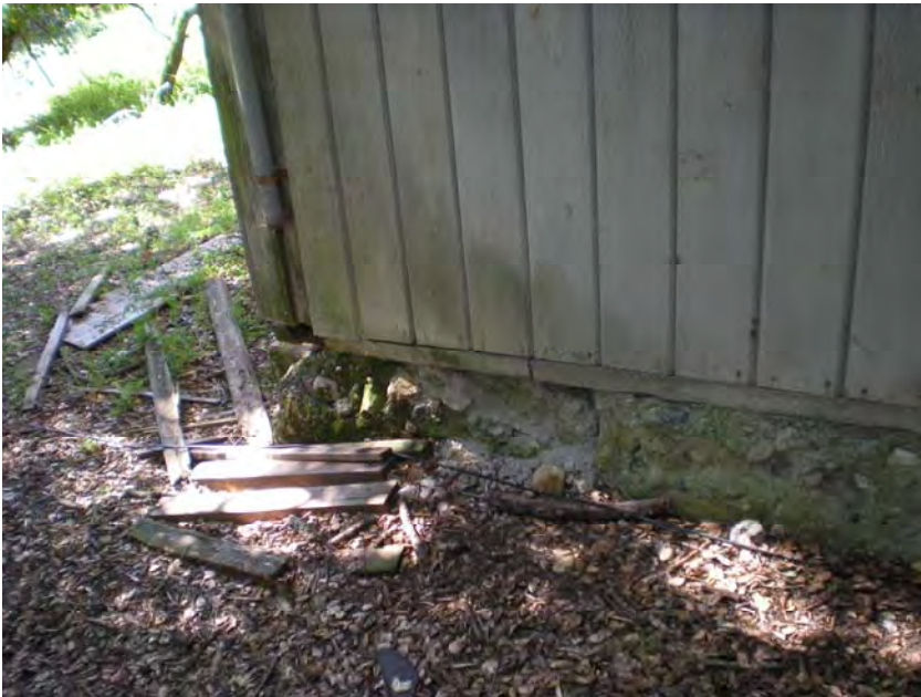
Image 111. Cottage, north façade, detail of east corner foundation.
