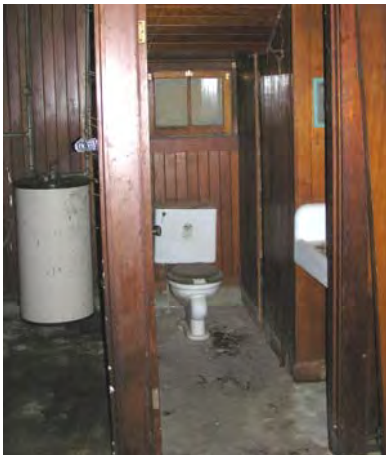
Image 87. Water Heater (left)
