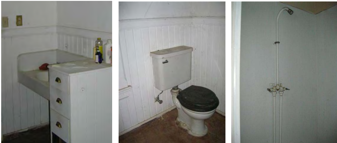
Image 45-47. Lavatory, Water Closet & Shower at Bathroom 109.
