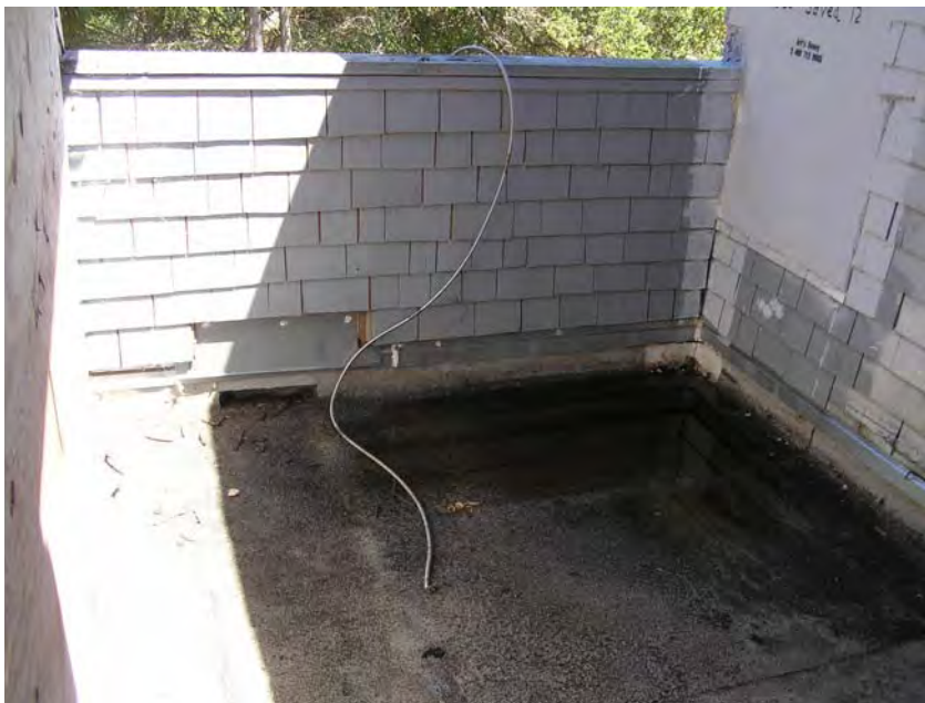
Image 16. Deck at second floor between Room 205 and 206, looking northeast.
