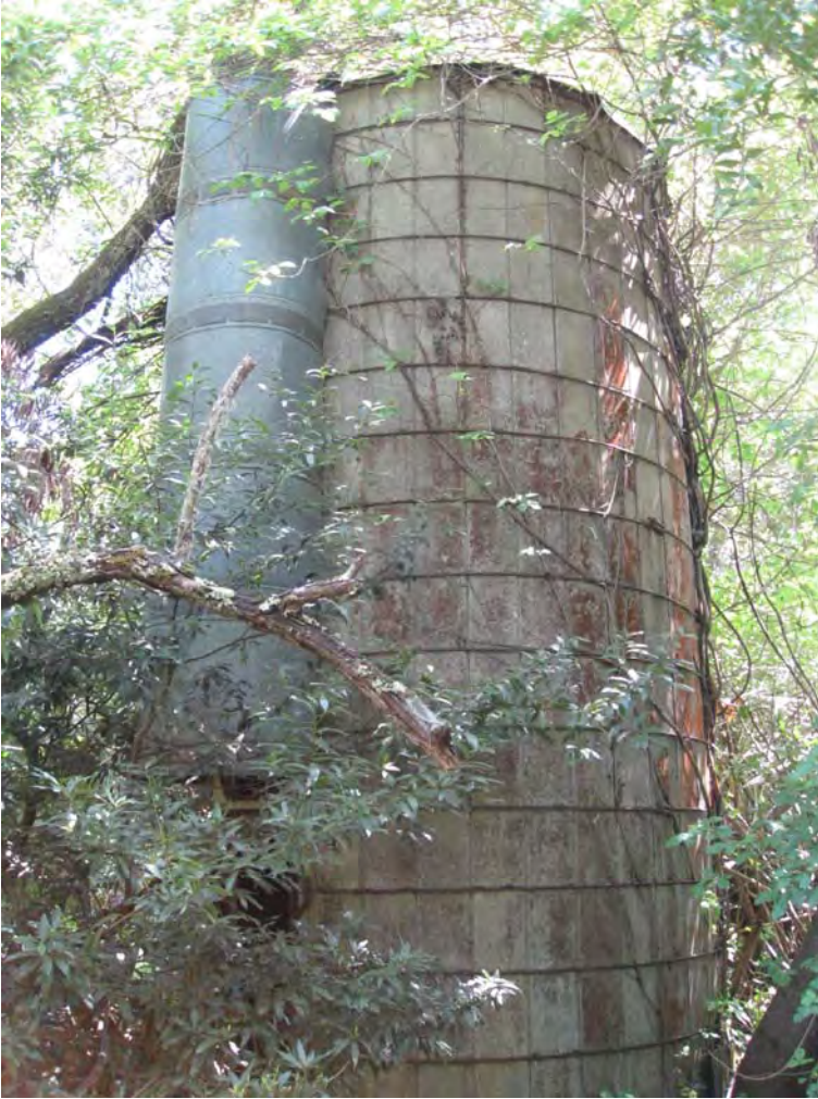
Image 136. Outbuilding, Silo west of barn, north side view of ladder enclosure.
