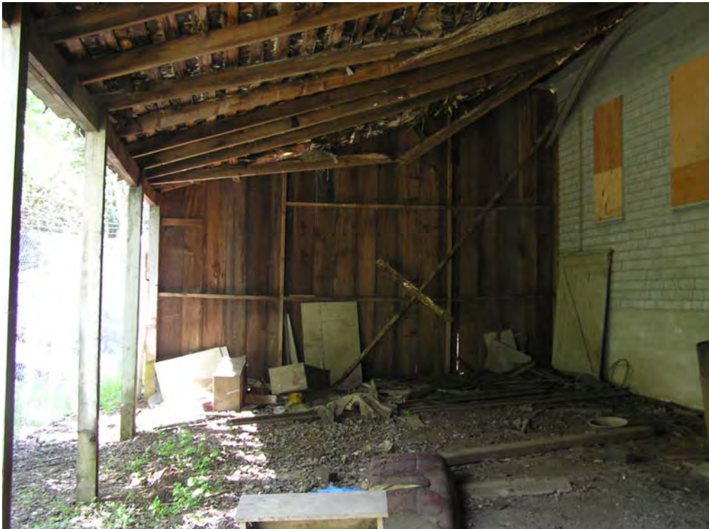
Image 81. Garage, lean-to addition at east side of building, view of collapsed roof.
