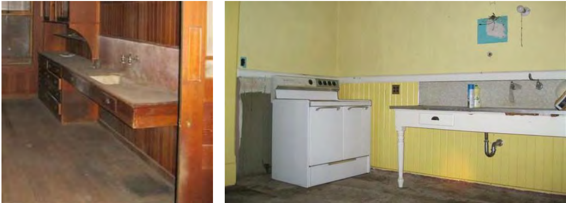
Image 48-49. Sink/Faucet at Kitchen 107 & Sink/Faucet at Kitchen 108.
