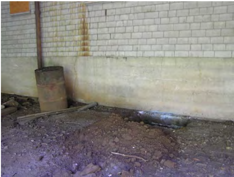
Image 72. Garage, concrete foundation at the east wall with vertical cracks and settlement.
