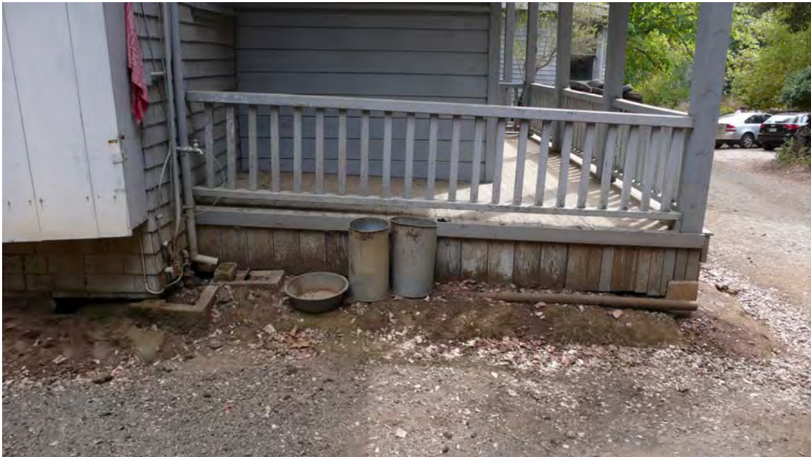
Image 33. Hawthorn House, southwest corner, damaged retaining structure at the corner of the building base (left) adjacent Porch 2, where siding is at grade.
