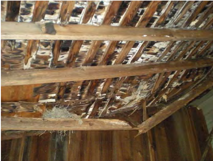
Image 82. Garage, east lean-to addition, detail of collapsed roof.
