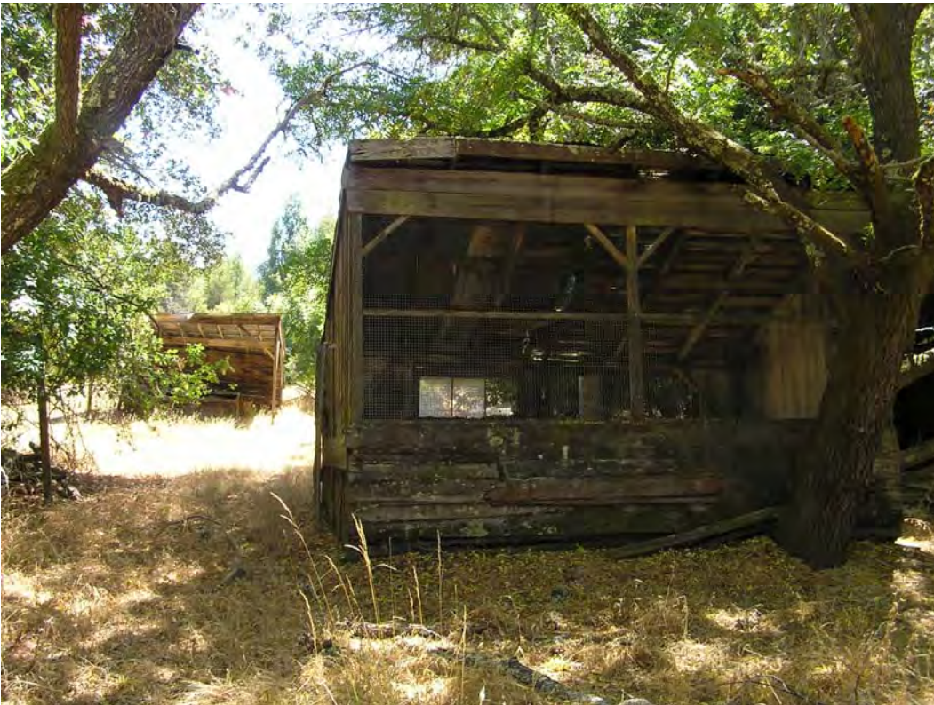
Image 133. Outbuildings, Raccoon Shed in foreground, Horse Shed in background.
