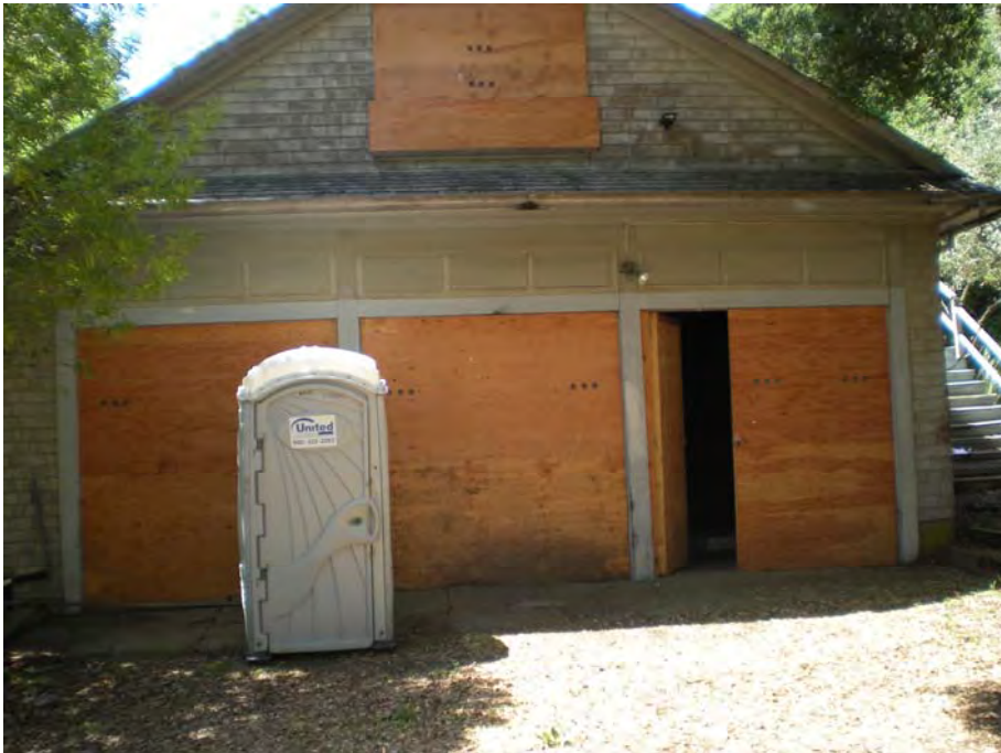
Image 84. Garage, north façade with three garage entryways.
