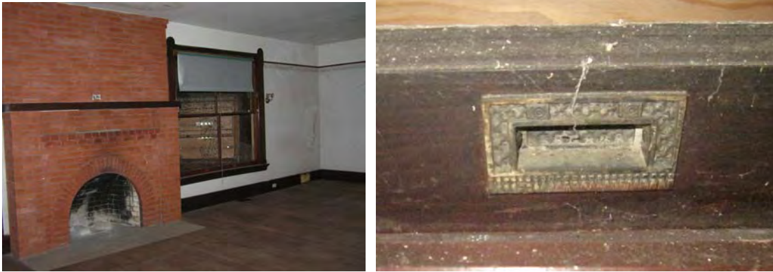
Image 19-20. Hawthorn House, Living Room 102, window and window sash lift.
