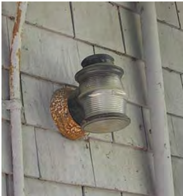
Image 96. Historic lantern fixture.
