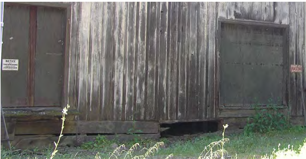
Image 124. Lower Barn, north façade, doorways are above grade, no foundations visible.
