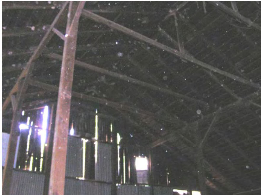
Image 126. Lower Barn, interior view of roof framing looking northeast.
