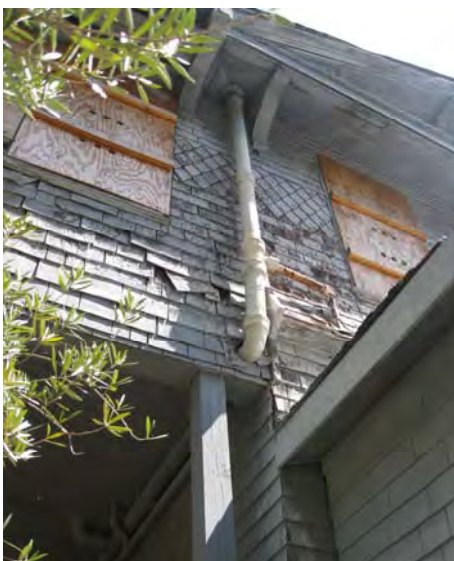
Image 7. Sewer lateral from second floor on west side of Hawthorn House.
