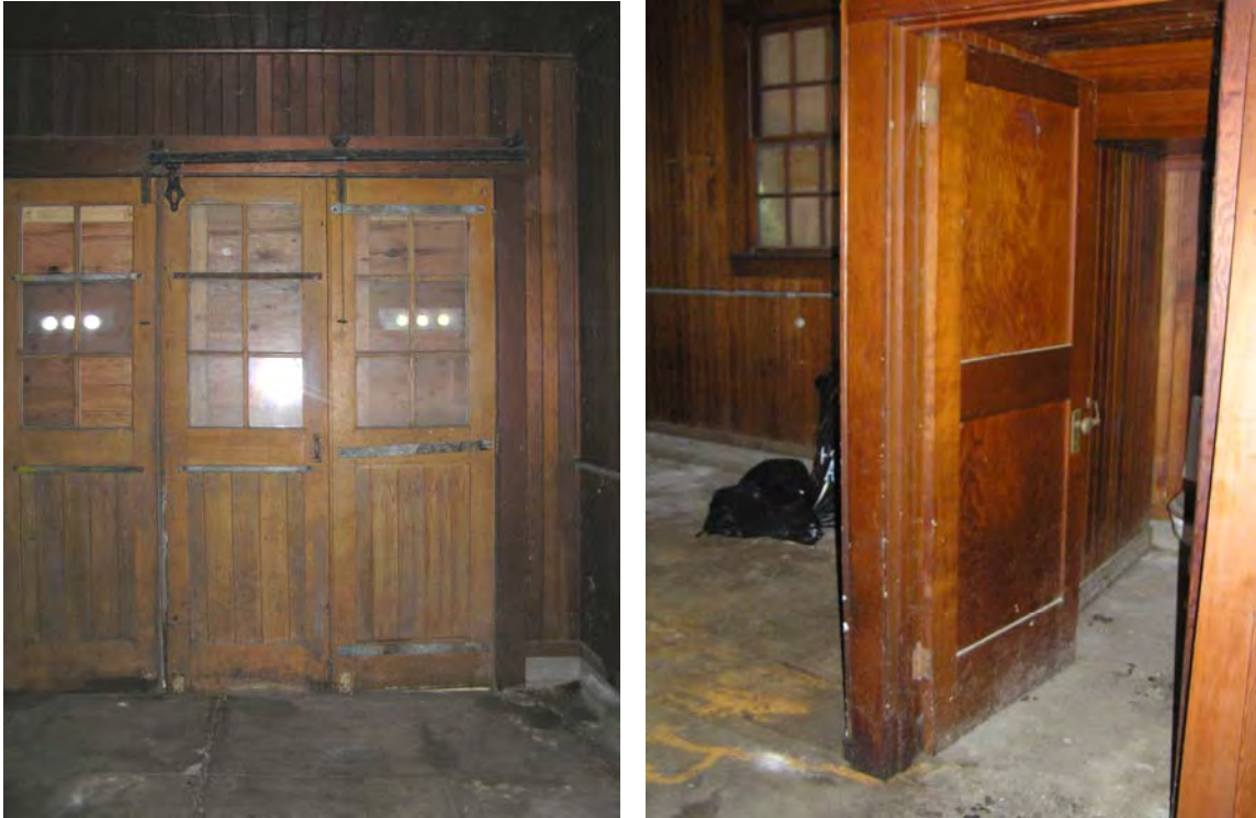
Image 73-74. Garage, interior view of garage door; window and toilet room door
