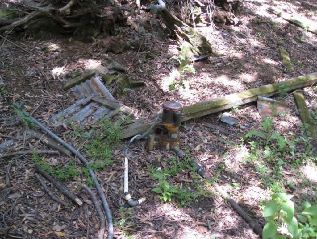
Image 12. Pump well head in wash area just north of the Lower Barn.
