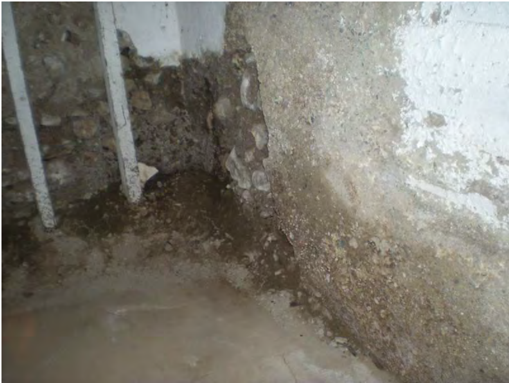
Image 38. Hawthorn House, corner east of basement entry.
