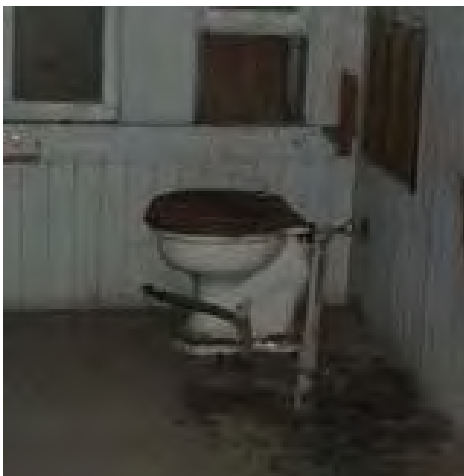
Image 55. Hawthorn House, Water Closet at Bathroom 304.
