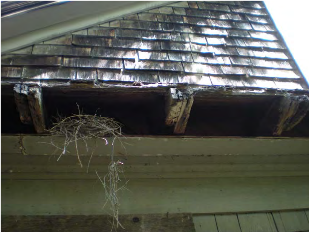
Image 85. Garage, south façade, detail of exposed rafters originally enclosed by eave and soffit boards, which should be rebuilt where missing.
