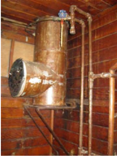
Image 86. Flue and Piping.
