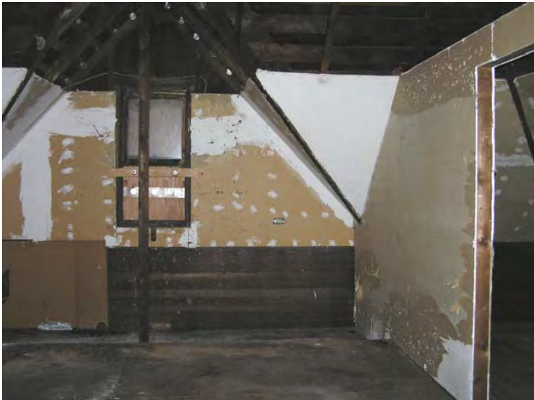
Image 110. Cottage, Attic framing partially finished with gypsum board.
