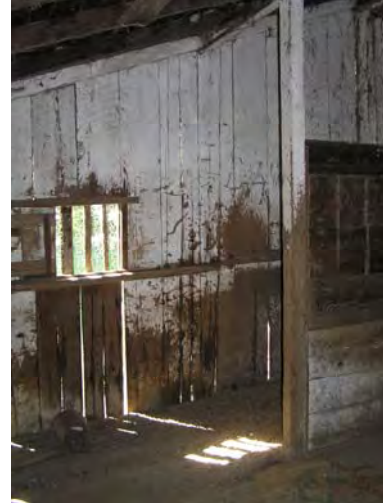
Image 122. Lower Barn, interior.
