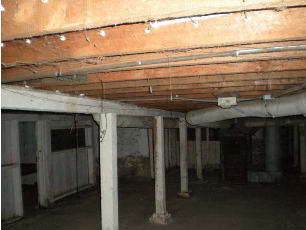
Image 34. Hawthorn House, Basement looking east.
