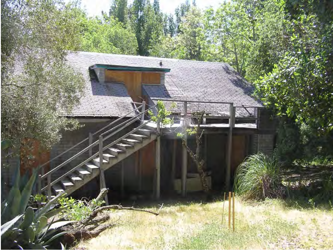
Image 71. Garage, west façade with stair to attic apartment.
