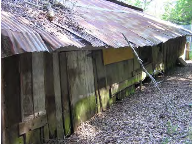
Image 121. Lower Barn, east façade.
