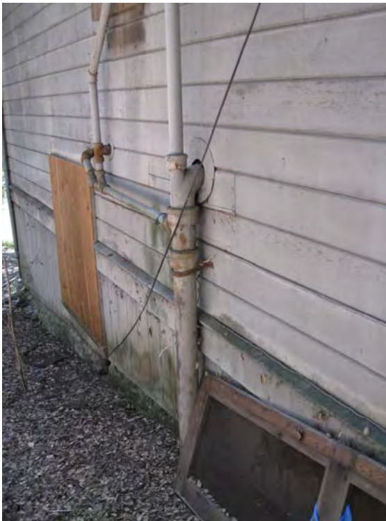
Image 8. Sewer lateral on east side of Cottage
