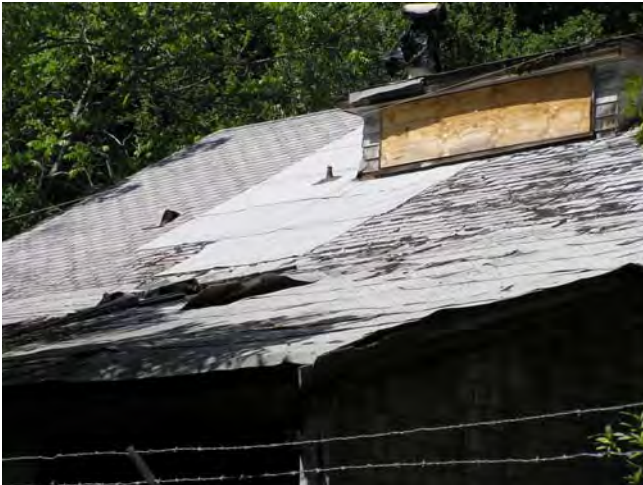
Image 79. Garage, deterioration at roof at east side (above).
