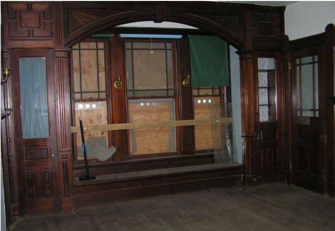
Image 25. Hawthorn House, Dining Room 104, decorative casework at south wall.
