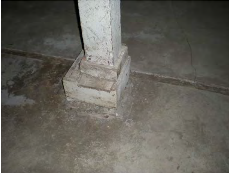
Image 36. Hawthorn House, post footing at main basement.
