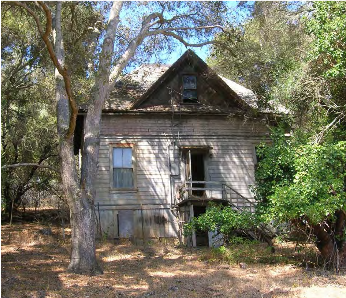
Image 104. Cottage, east façade.
