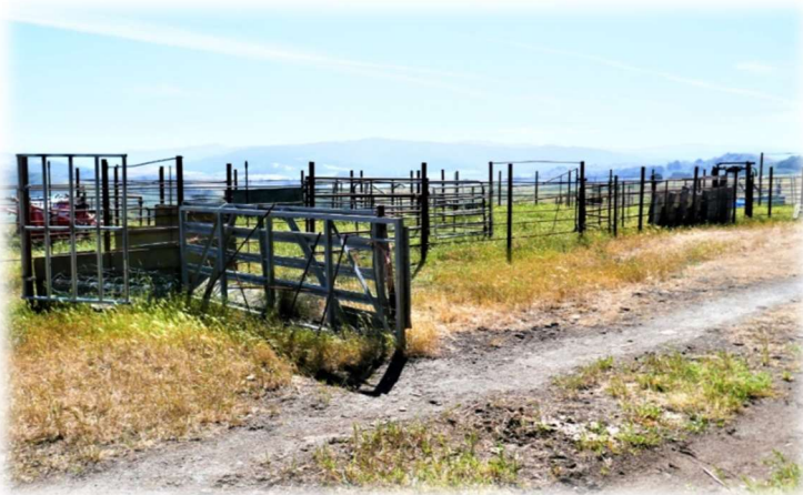
Figure-14: The corral located on the western side of the Butano Farms grazing unit is small and poorly constructed. The corral is usable but not reliable to efficiently process, ship or receive cattle. The corral has been pieced together over the years with a variety of different gates and panels.
