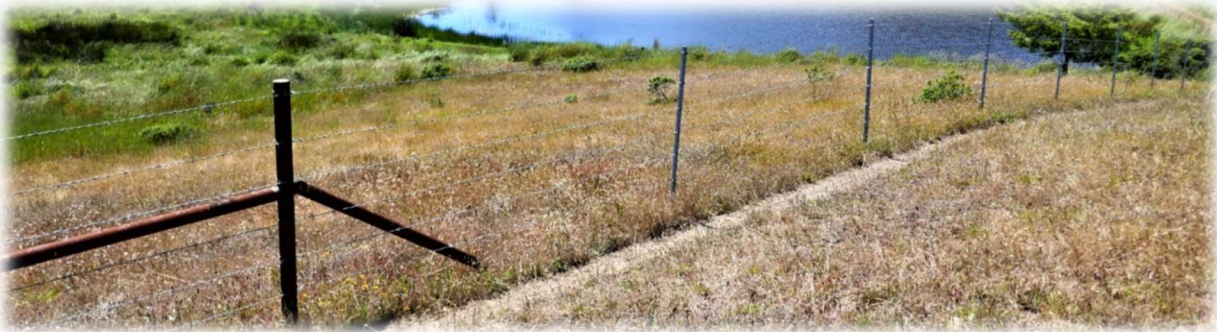
Figure-19: Recently installed fence on the Goat Ranch grazing unit using steel braces posts and t-posts.
