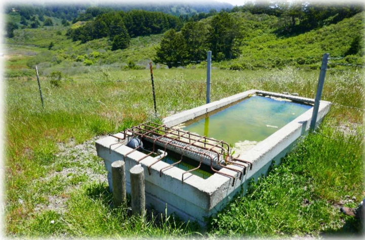
Figure-16: (left) A water trough near the eastern edge of the Holm Ranch grazing unit. The trough is supplied via water pumped from the well on the ridgetop to the west.
