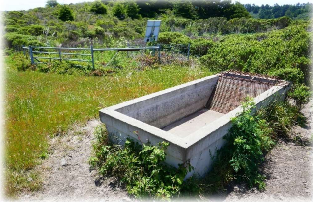
Figure-17: (left) A concrete water trough adjacent to a stockpond. The solar panel (center of photo) powers a pump in the pond which sends water to the trough. Three similar systems are present in the Hidden Springs grazing unit. Under recent drought conditions all ponds have failed to maintain an adequate water supply to keep the troughs full.
