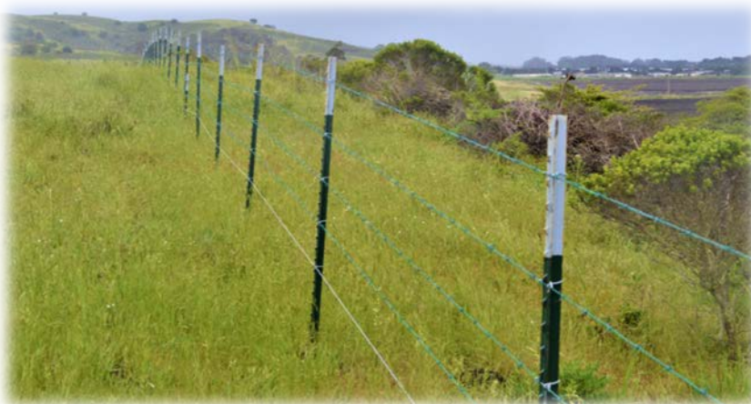
Figure-8: Recently installed barbed wire fence along the western border of the Ranch. The perimeter of the Ranch is considered “cow tight” with a combination of new barbed fencing and older barbed wire fence in fair condition.
