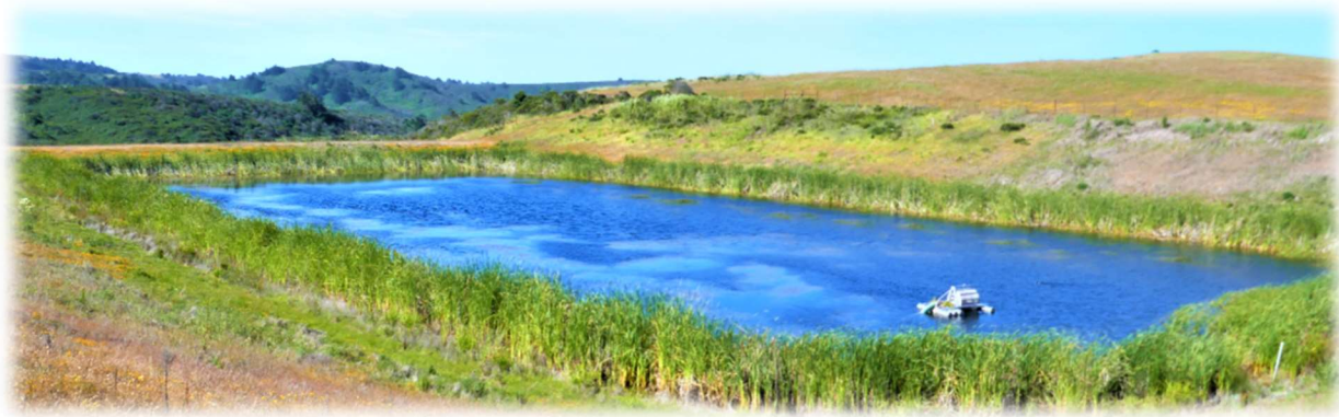
Figure-8: Developed reservoir on the Butano Farms property used primarily for irrigating local farm fields. Note the floating solar pump in the water which supplies stockwater to nearby storage tanks and troughs.
