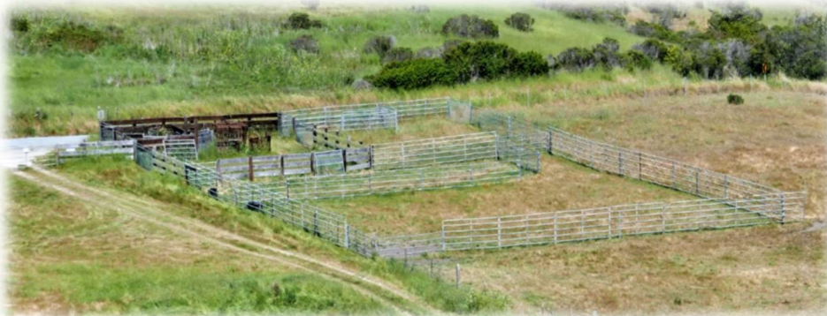
Figure-15: Corral on the Goat Ranch grazing unit. Corral consists primarily of panels owned by the current grazing tenant.
