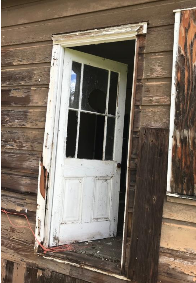
Some vandalism on door frame
