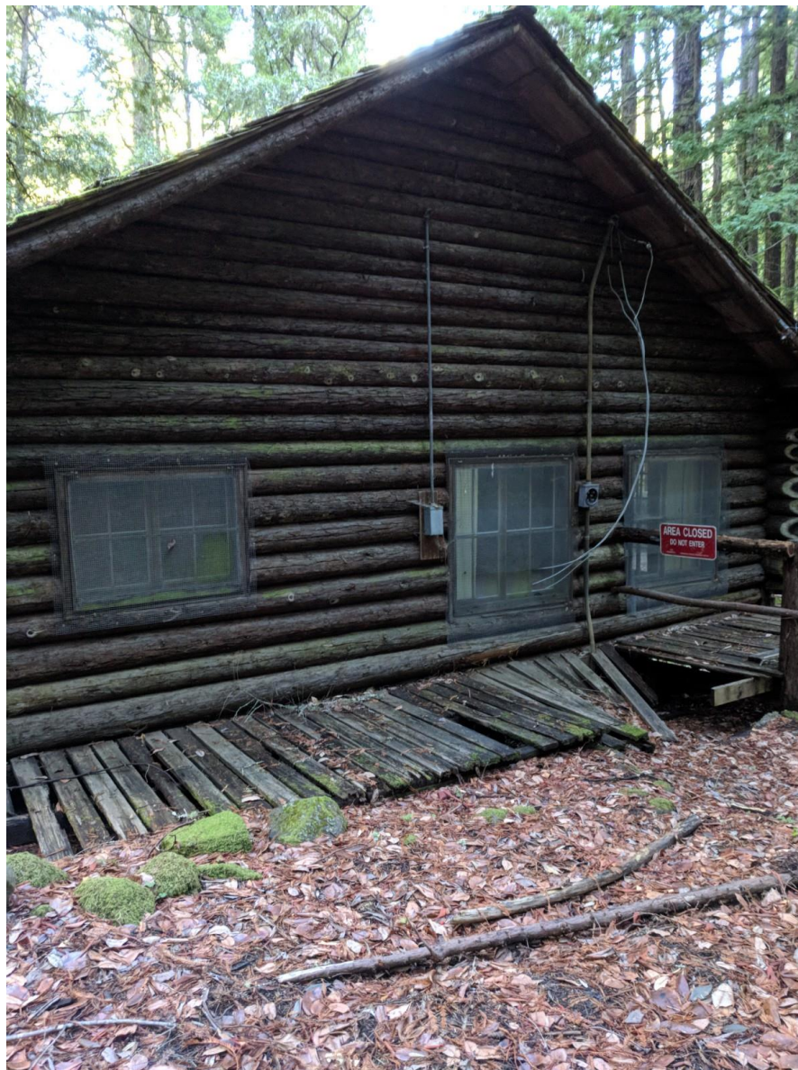
Deteriorated deck around the cabin
