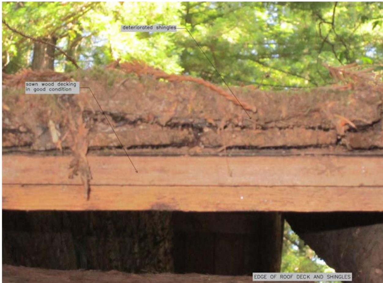
Deteriorated roof shingles
