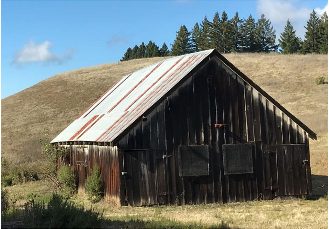
Some rust on roof
