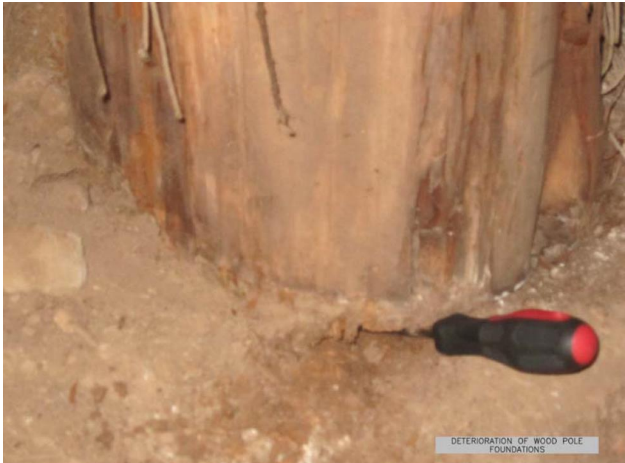
Deteriorated vertical pole foundation
