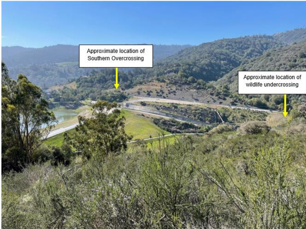
Figure 2.2.3-2: View of the southern and central project area, looking west/southwest from the Jones Trail; yellow arrows indicate approximate locations of the Southern Overcrossing and wildlife undercrossing
