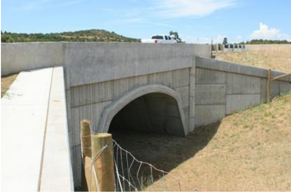
Figure 1.4-3: Example of a precast arch wildlife undercrossing with wingwalls and directional fencing, at U.S. Highway 160 in southern Colorado (Muller Engineering Company 2022)
