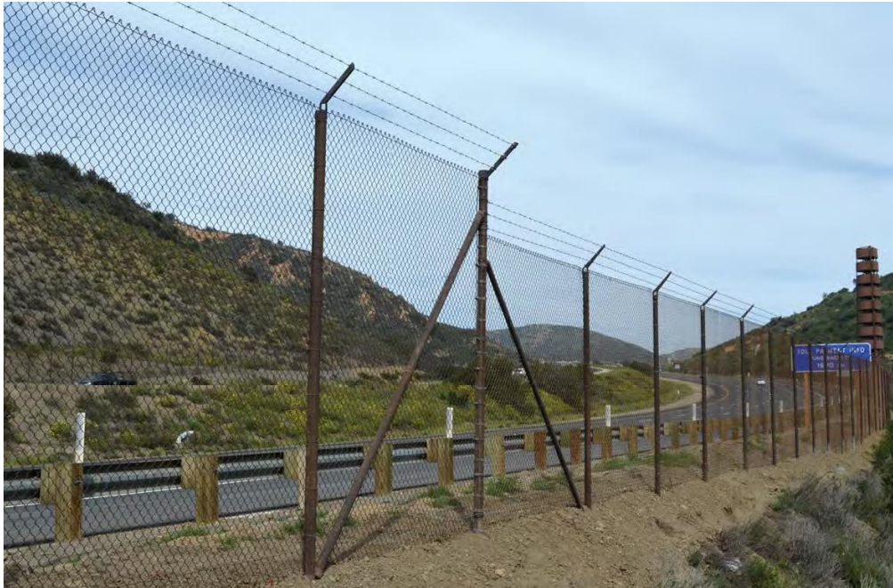
Figure 1.4-5: Example of wildlife fencing along SR 241 in Orange County, CA (McFall et al. 2015)
