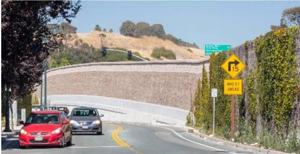
Figure 1.4-7: Example of a masonry sound wall on top of a concrete barrier, El Portal Drive, San Pablo, CA (AECOM 2020). The height, color, and materials used for this project may differ
