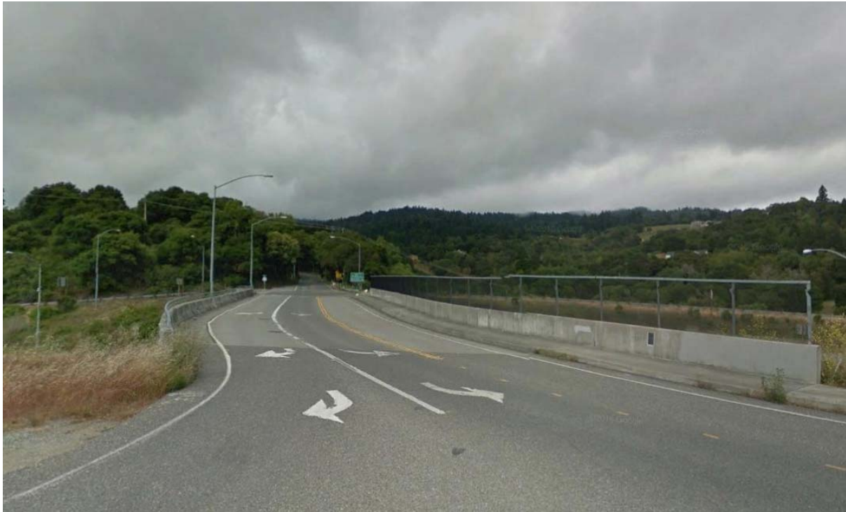
Figure 13: Bear Creek Road/Alma Bridge Road Overcrossing
