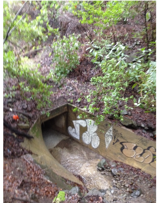
Existing culvert inlet on west side
