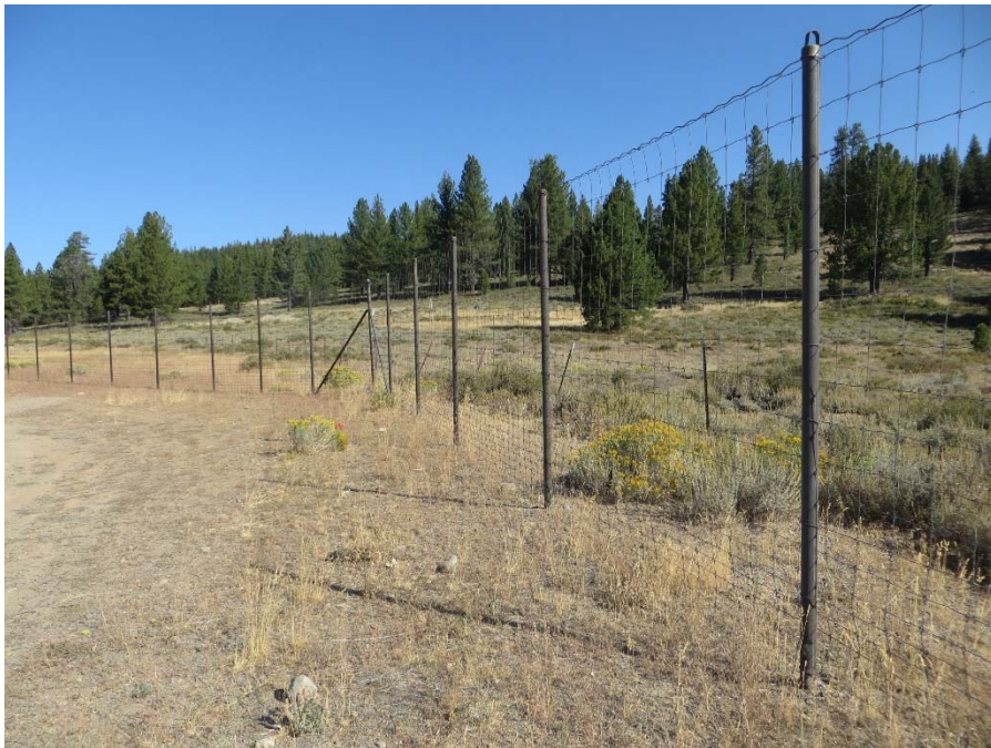
Photo 1: Example of directional fencing associated with a wildlife crossing on Highway 89 in Northern California
