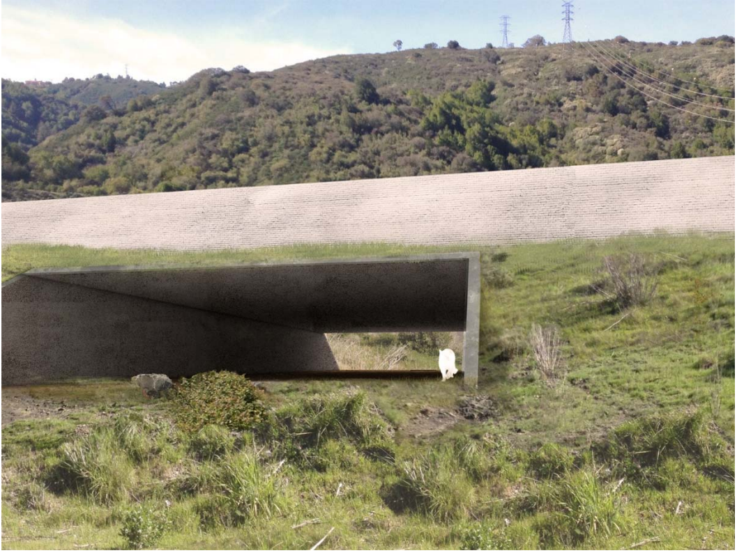
Figure 11: Photo-Rendering of Trout Creek Wildlife Undercrossing, before & after
