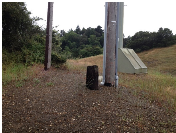
View of east landing area looking south west – note utilities and cell towers
