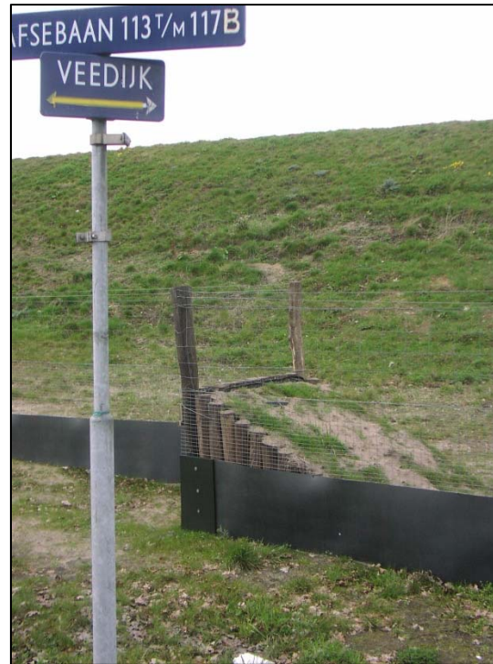
Example of fencing to direct small animals to a wildlife crossing in the Netherlands
