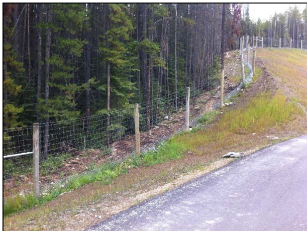
Example of directional/exclusion fencing – wire at top is to help deflect falling branches
