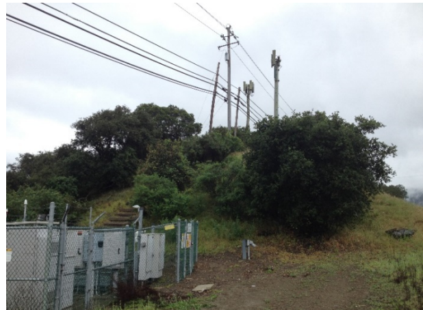
View from east side south toward potential landing area – note utilities and cell towers
