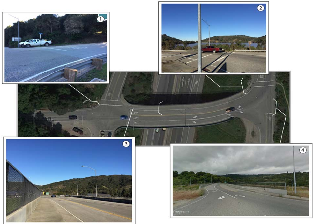
Figure 32: Bear Creek Road Overcrossing Existing Conditions
