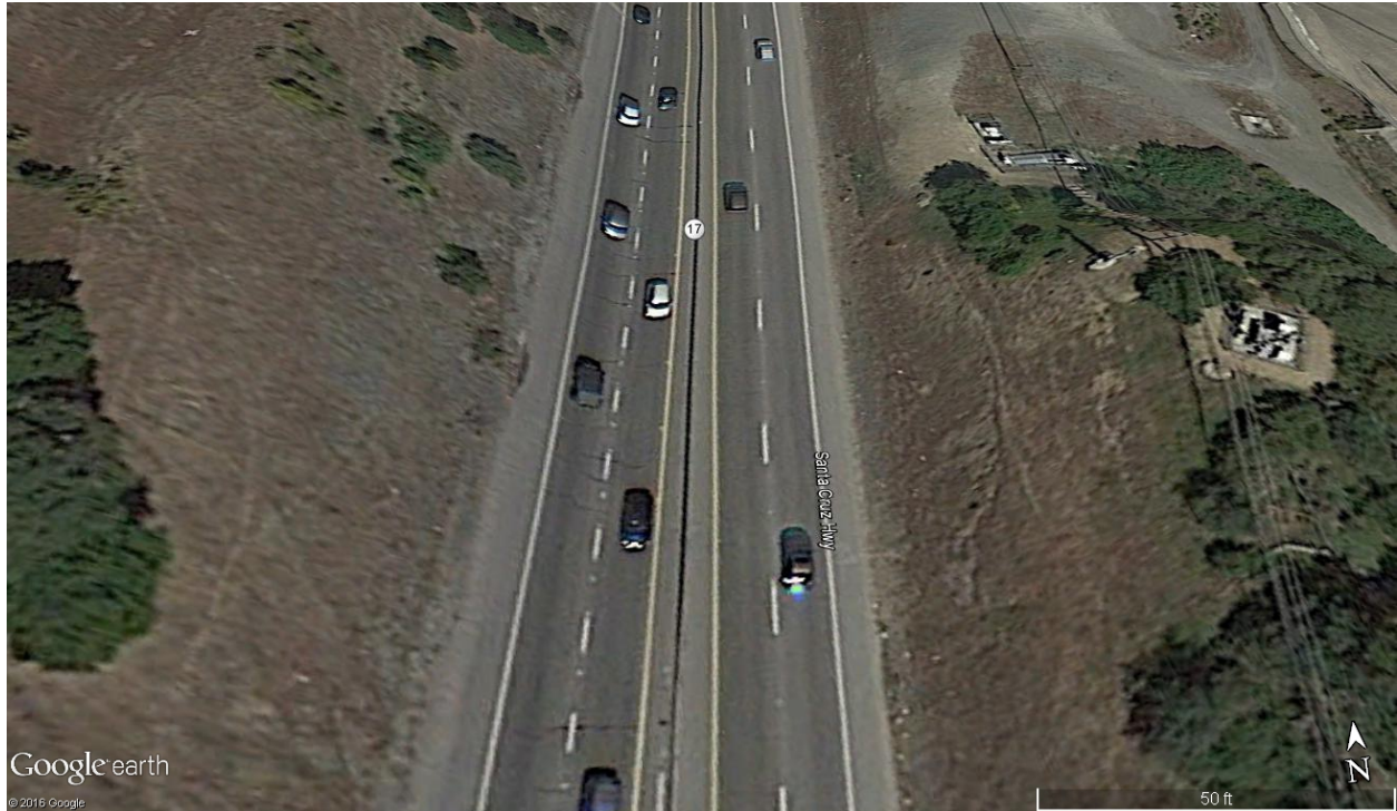
Potential overcrossing site looking north
