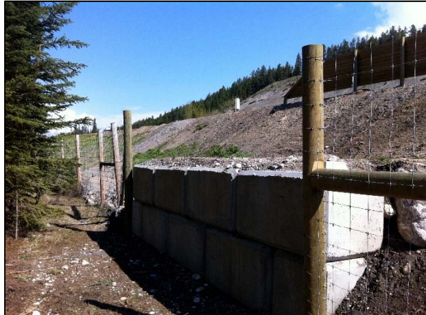
Example of wildlife “jump out” to allow escape from highway
