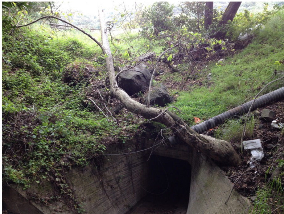
Figure 4: Ravine Culvert Inlet
