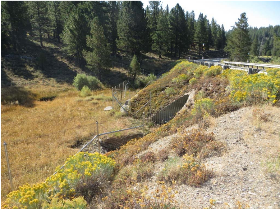
Photo 2: Directional fencing leading to a culvert on Highway 89 in Northern California
