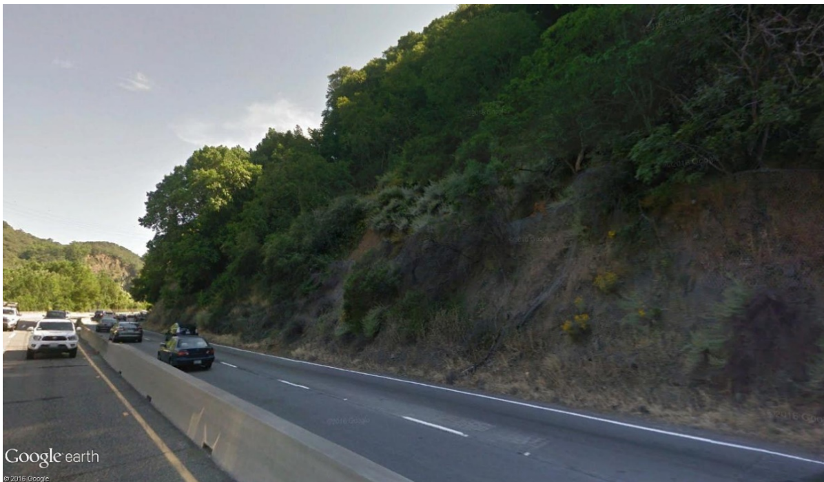
Figure 26: Eliminated Alternative 6, looking south, view of steep hillside where potential undercrossing would exit
