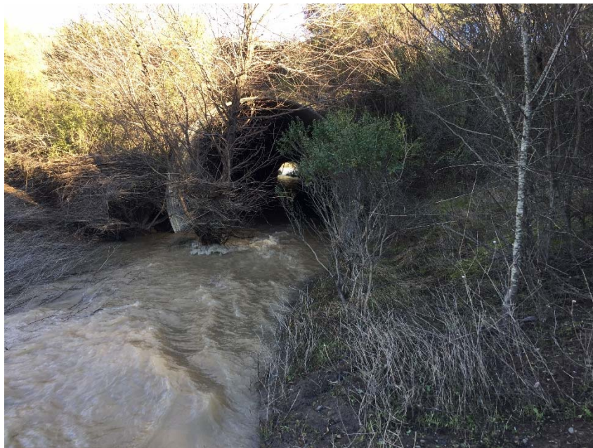
Figure 10: High water flowing through Lexington Culvert (January 13, 2017)
