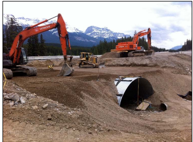
Example of wildlife undercrossing under construction in Banff N.P. Alberta
