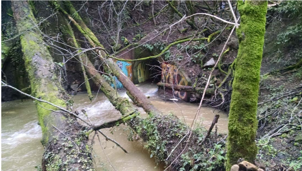
Photo 4: Aldercroft Culvert, Looking West During Wet Conditions
