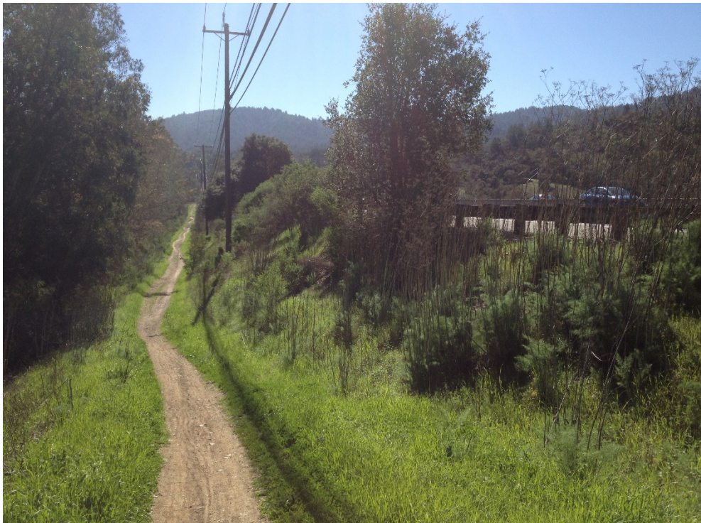
Potential undercrossing opening location – east side
