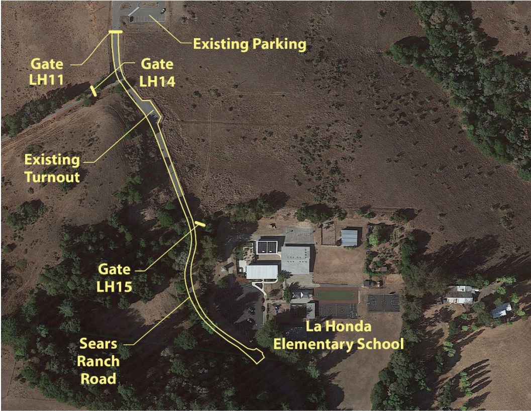
Site B2 - Sears Ranch Road Widening
