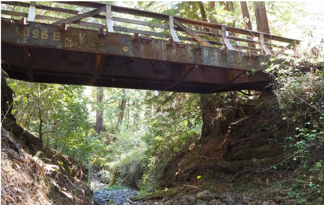
Figure 2-Br-2 Site D Bridge over La Honda Creek facing west
