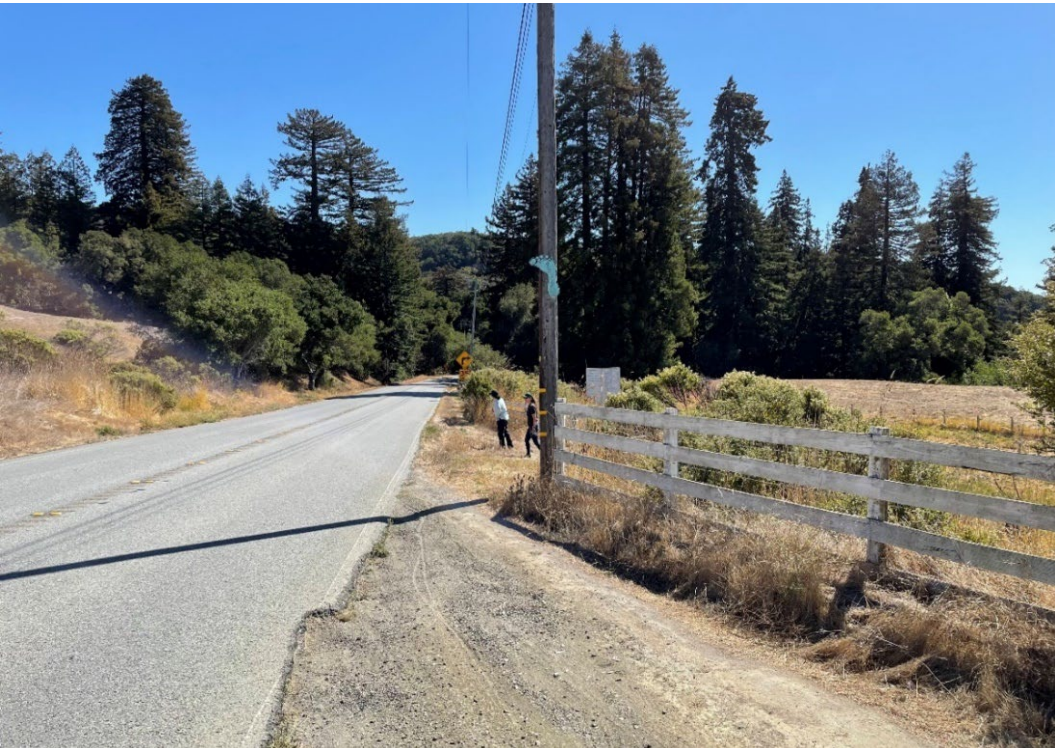
Figure 3-E3-13 Site E3 existing exit drive at Preserve Gate RED01 facing southbound on SR-84
