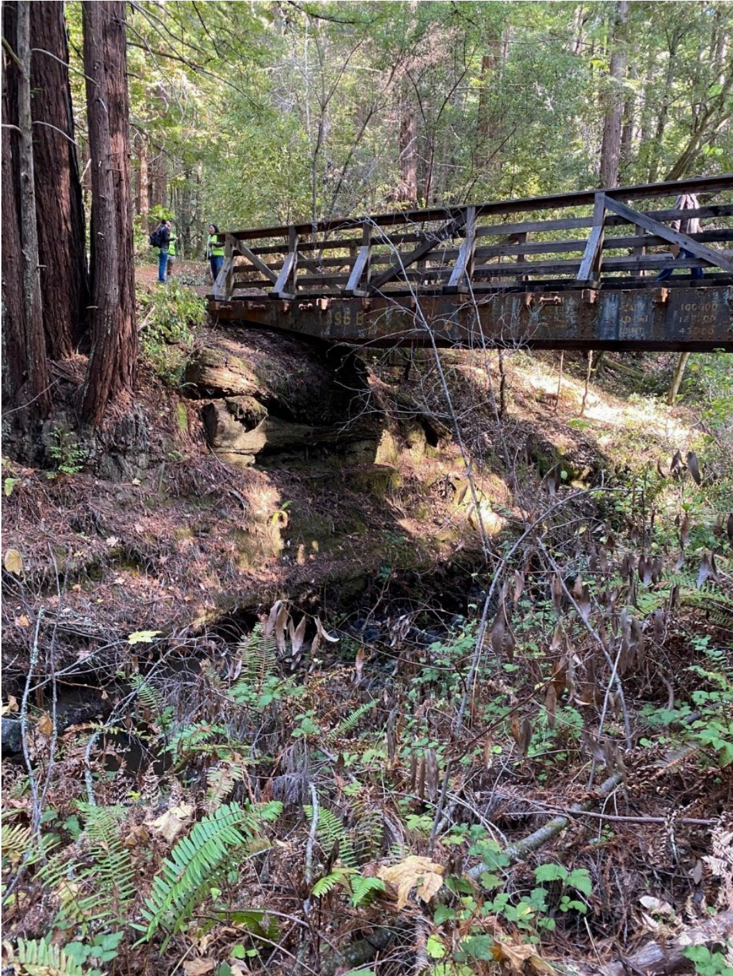
Figure 3-Br-3 Bridge over La Honda Creek at Site D facing east
