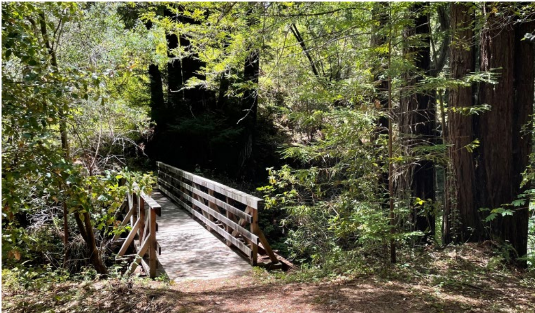
Figure 3-Br-1 Bridge over La Honda Creek at Site D. Also see Figures: 4.1, 4.2, and 4.3
