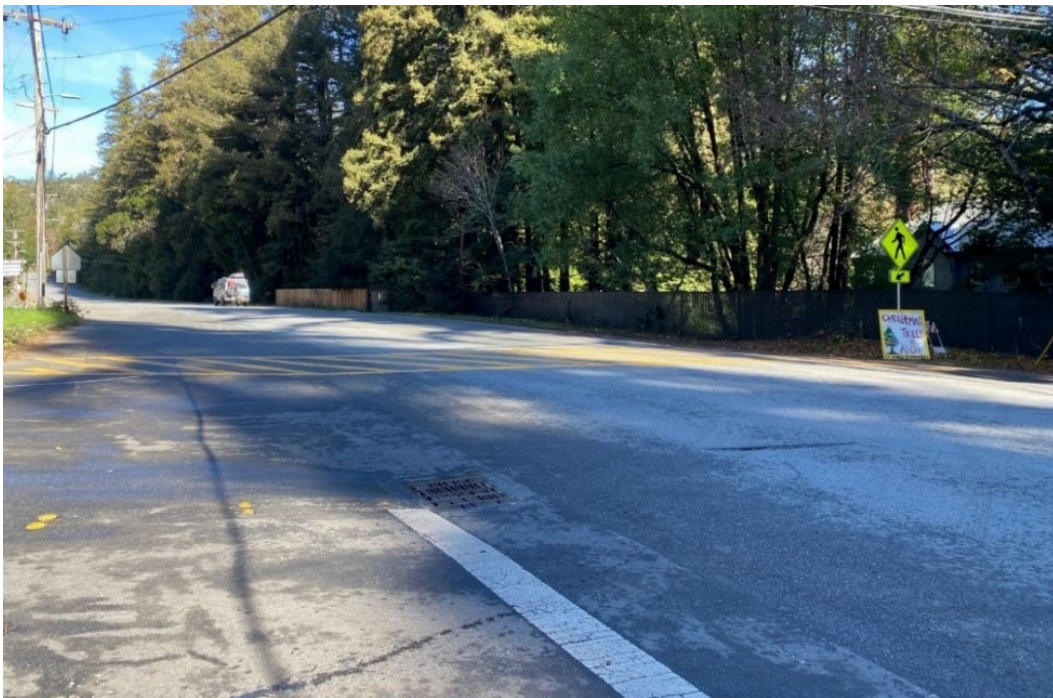
Figure 3-B2-5 SR-84 at Sears Ranch Road facing north
