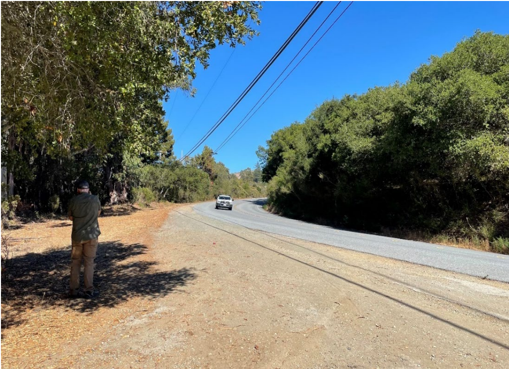
Figure 3-D-4 Site D facing north at SR-84
