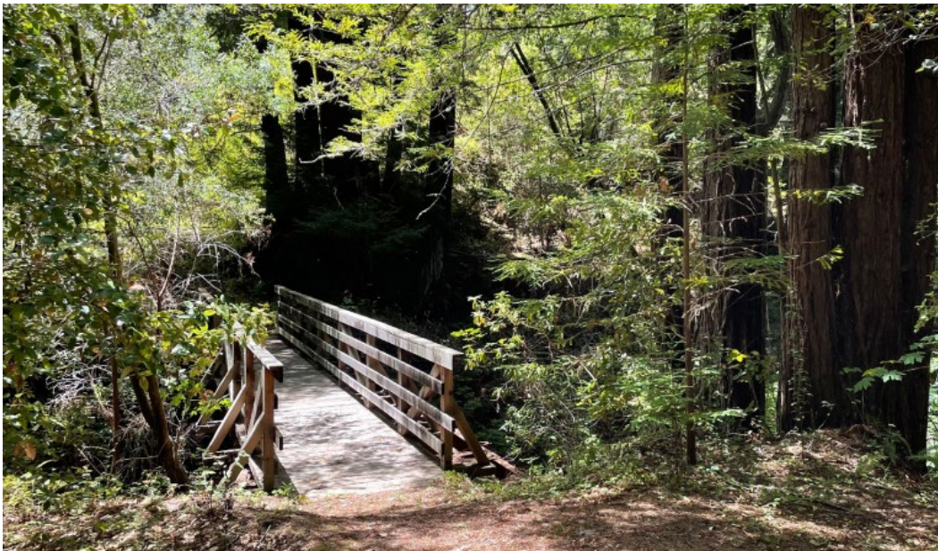
Figure 2-Br-1 Site D Bridge over La Honda Creek that connects Site D to the Preserve trail/ranch road network.
