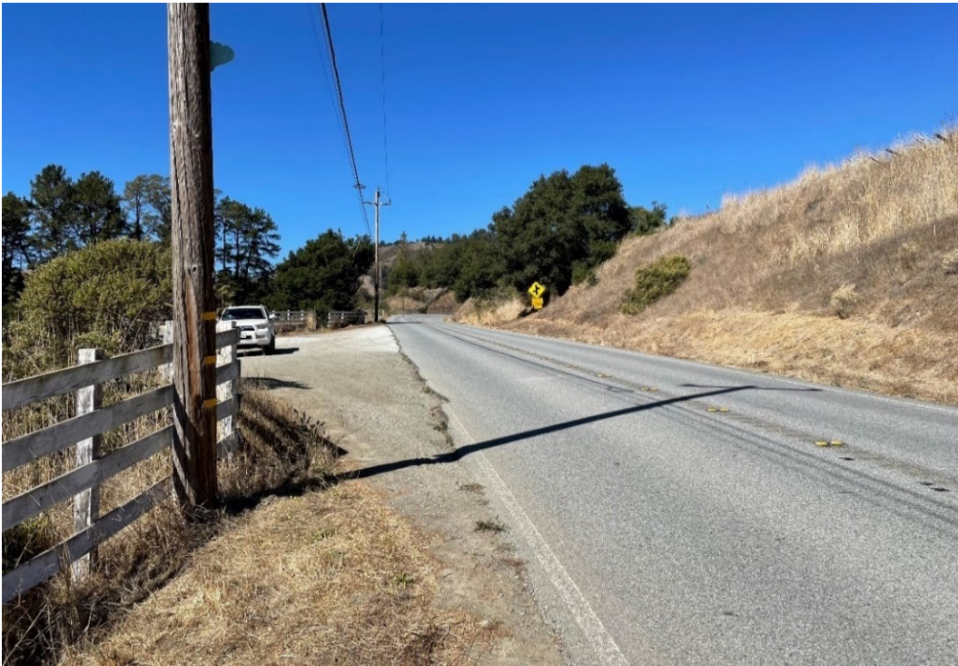
Figure 3-E3-12 Site E3 existing exit drive at Preserve Gate RED01 facing northbound on SR-84
