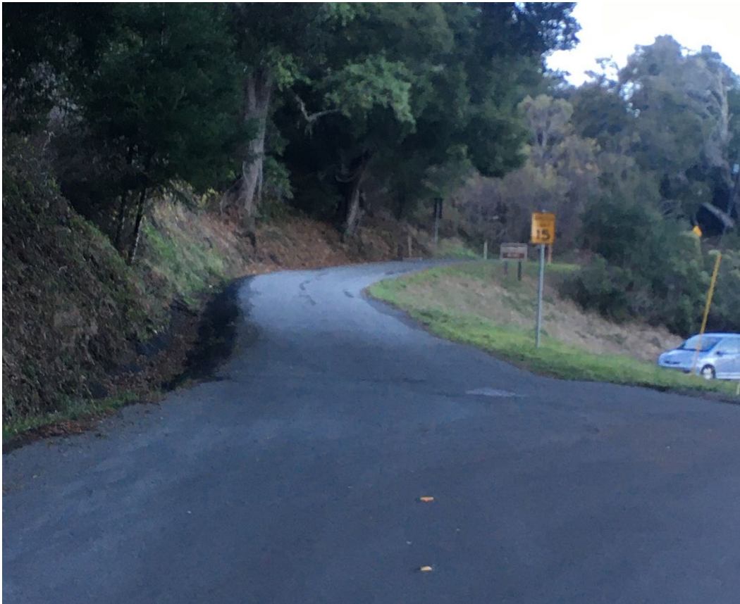
Figure 3-B2-8 Sears Ranch Road facing north at narrow section of road near school
